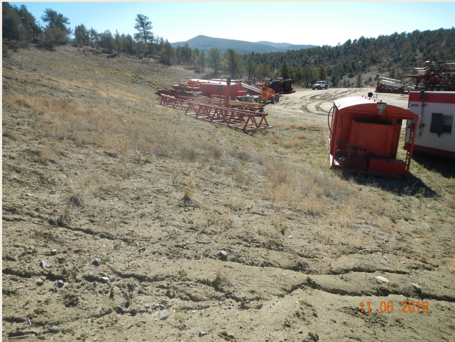
Photo 4. View of the eastern project area from the northeastern corner facing southward. Drilling equipment remains on location. Rilling is occurring in several areas along the cut-slope. Poor vegetative cover here. Some desirable species such as Indian ricegrass ( Achnatherum hymenoides ) and western wheatgrass ( Pascopyrum smithii ) observed. However bare ground and weeds such as Russian thistle ( Salsola tragus ) dominate.
