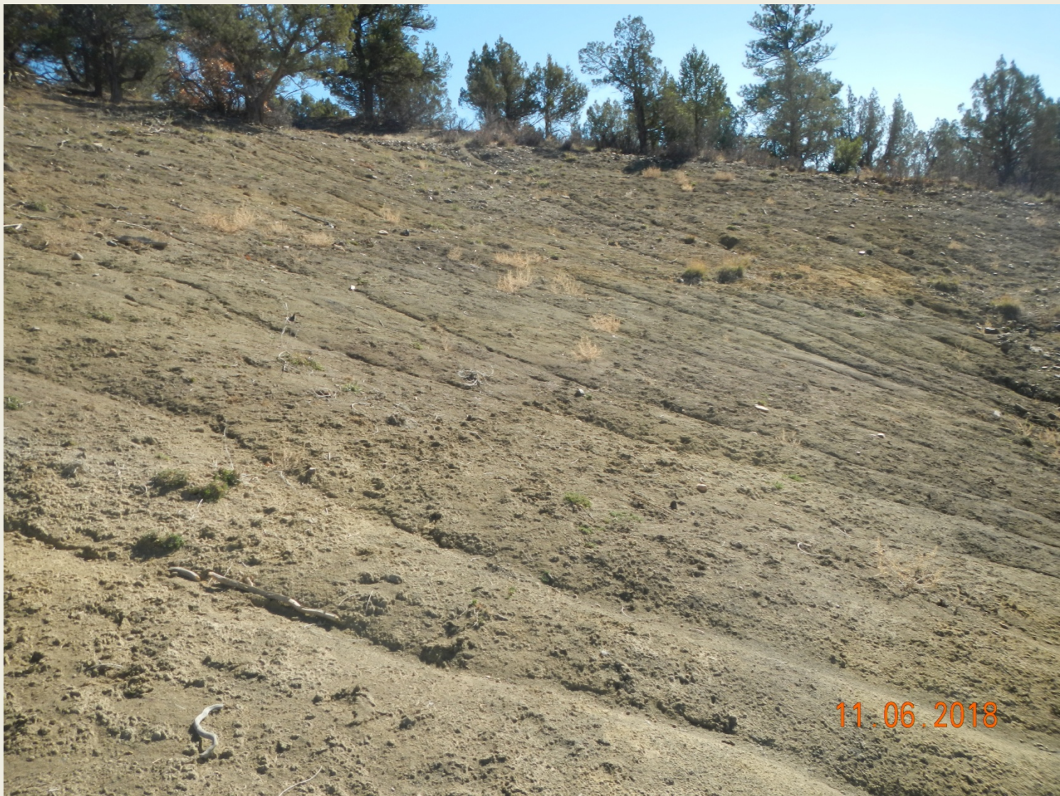
Photo 5. View of the southeastern cut-slope. Poor revegetation and rilling is occurring throughout.
