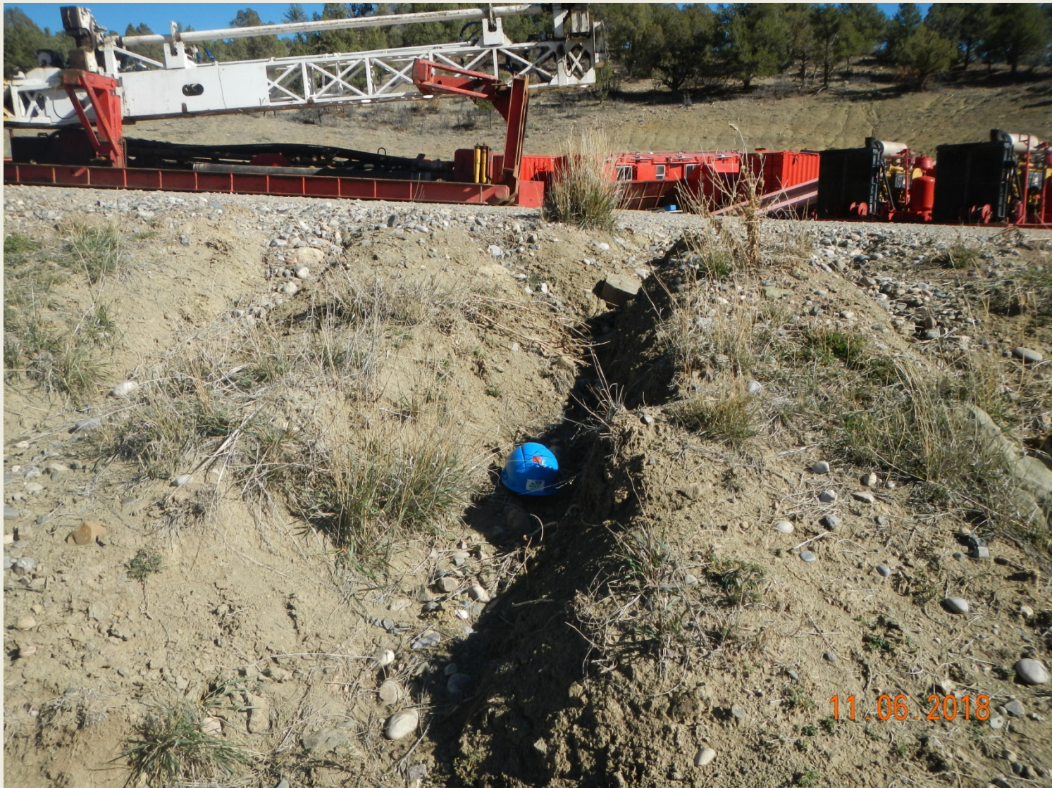
Photo 2. View of erosional channel approximately 1.5 feet wide and deep within the western project area.
