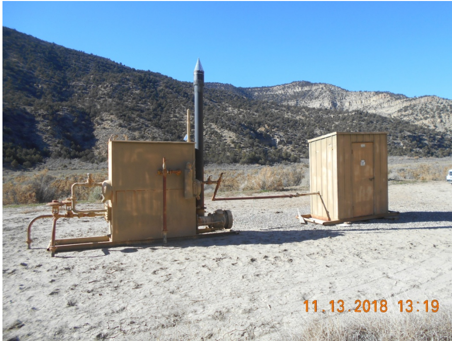
Separator and Meter housing
