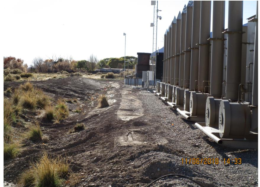
Debris along berm has been removed. Straw bales have been re-installed as needed. Holes behind separators have been filled in. Weed debris has been cleared from diversion ditch and berm.
