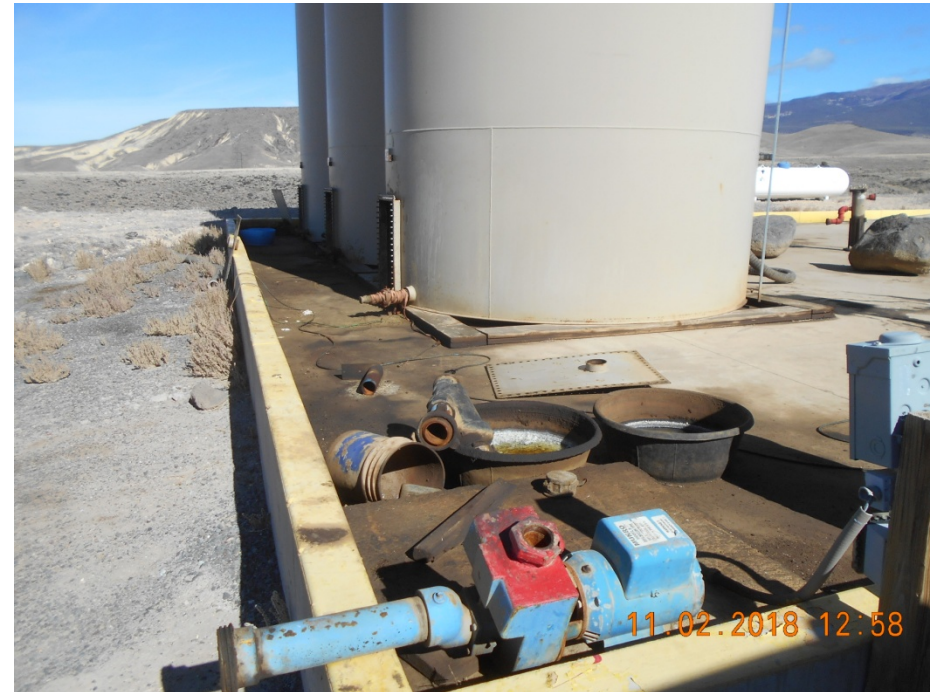
SW corner looking N of cement bermed offload pad. 3-400 bbl tanks with access hatches removed.
