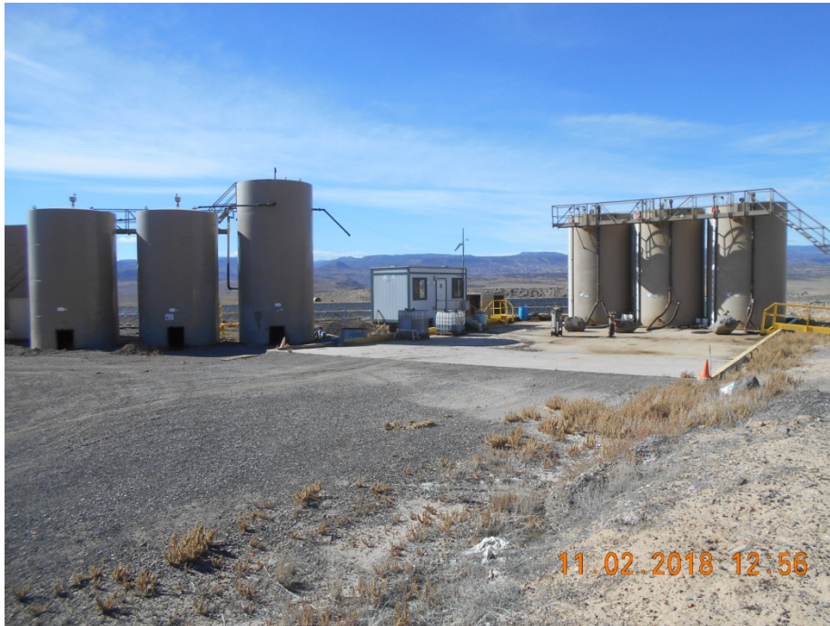
Overview of water disposal facility looking SW. 2-400 bbl and 1-500 bbl tanks. Access hatches removed. 3-400 bbl tanks with cement bermed offload pad.
