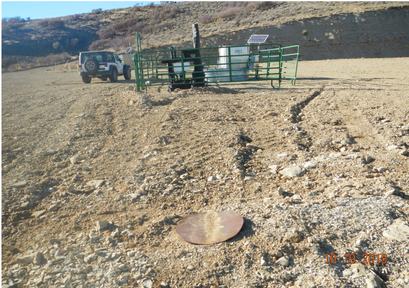
Photo#1: View of Plate covering Casing; following photo shows uncovered.
