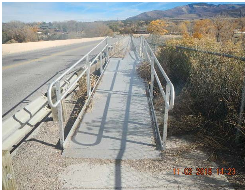
Poly pipe crossing Colorado River on CR 301. Walk Way installed over Poly pipe.
