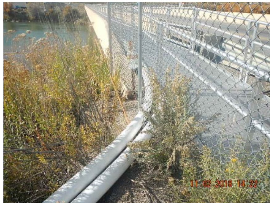
Pipe leaving CR 301 Bridge to cross under bridge and re route to the east side of CR 301
