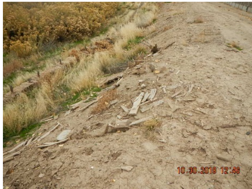
Debris incorporated into the un stabilized berm
