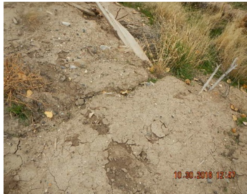
Berm not stabilized with signs of erosion.
