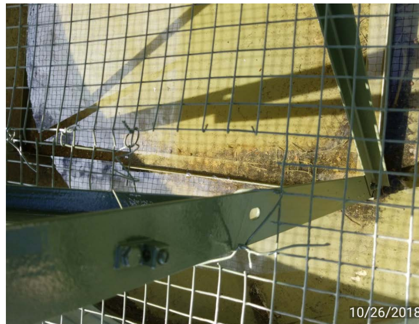
Hole in mesh in Methanol secondary containment. Birds can fly in, but can't fly back out.
