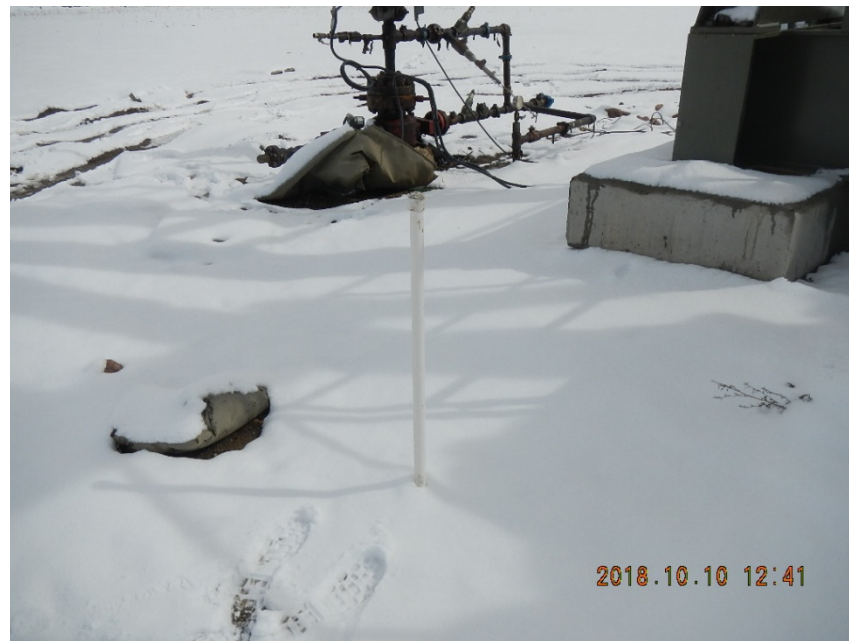
One-inch PVC riser pipe and insulation beneath snow.
