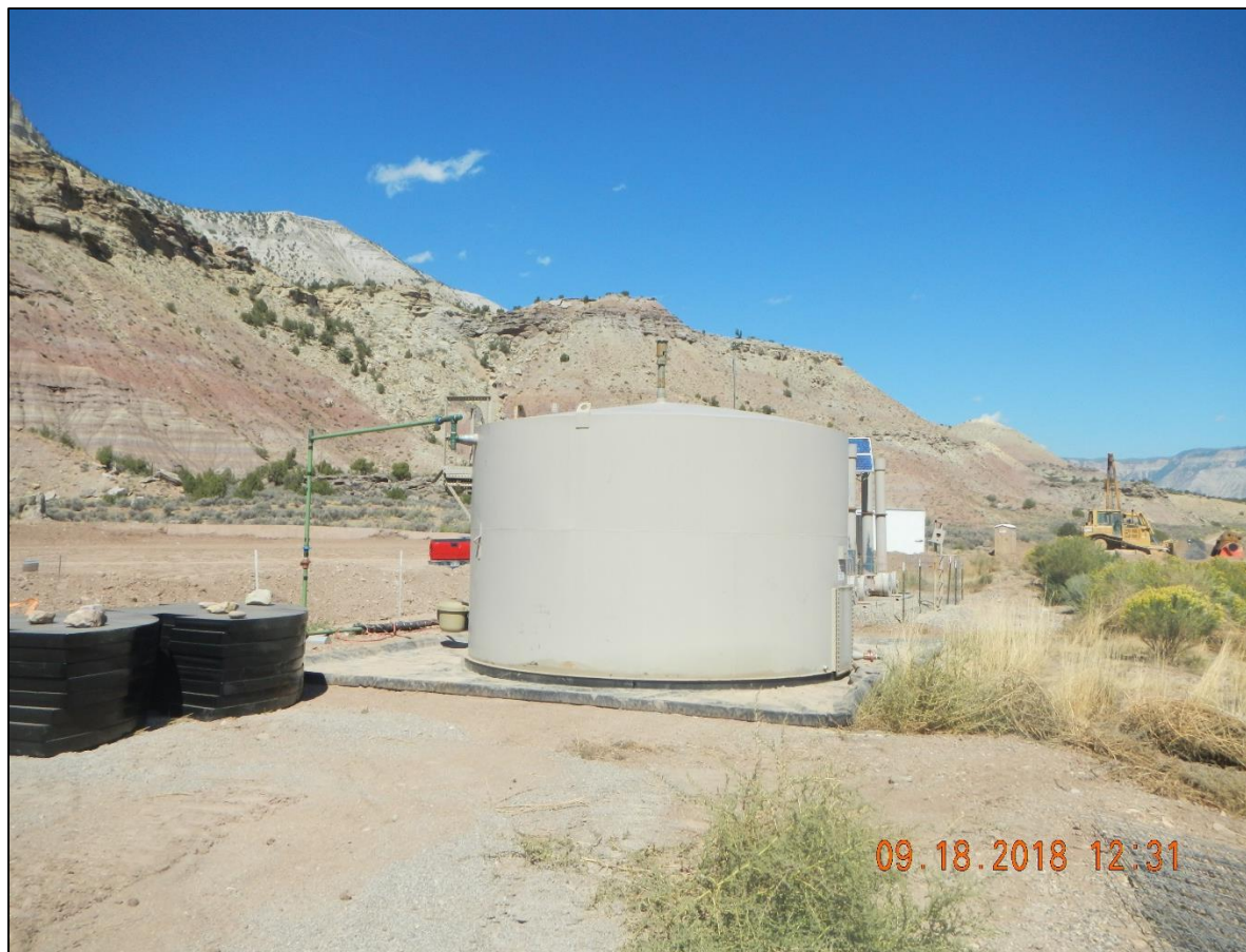
Dead weed debris. Inadequate containment for tank.
