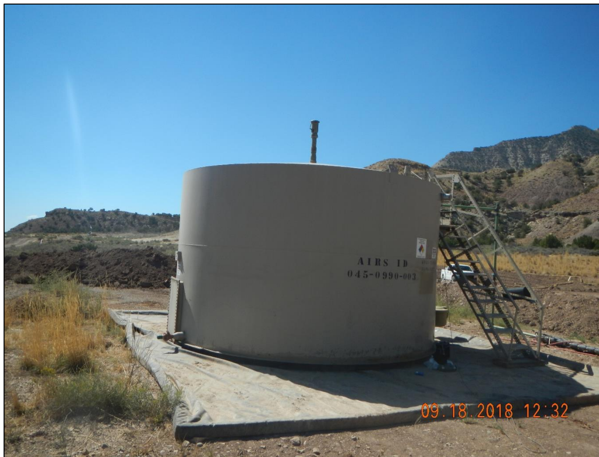
Dead weed debris. Inadequate containment for tank.
