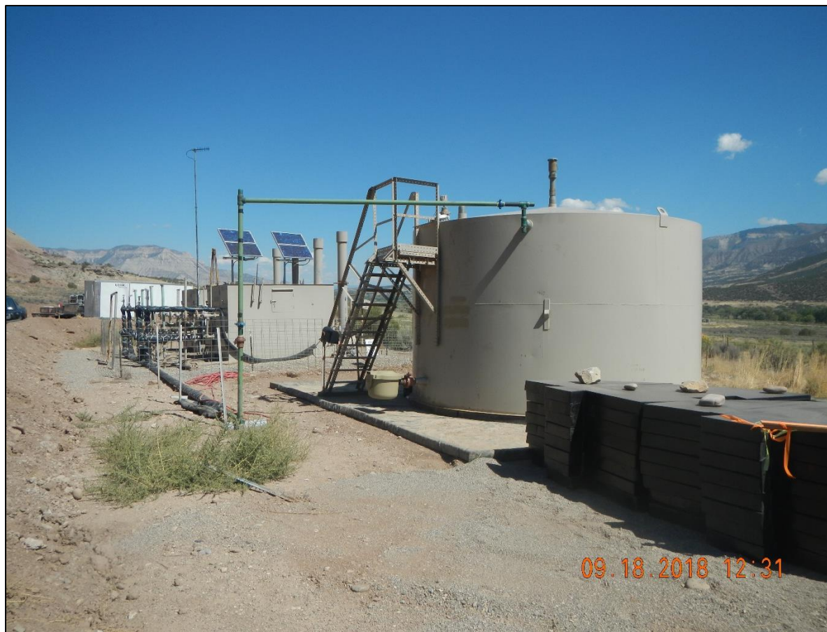
Dead weed debris. Inadequate containment for tank.
