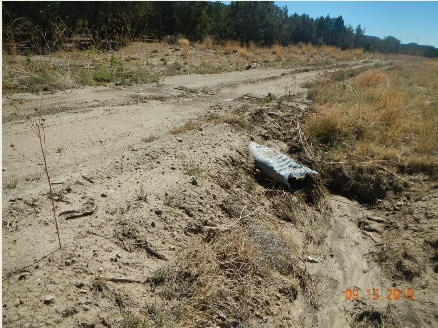
Photo 6. View of area along the access road where culvert is blocked on upstream side and stormwater flows over the road surface resulting in erosion on the road and where it flows into the drainage.
