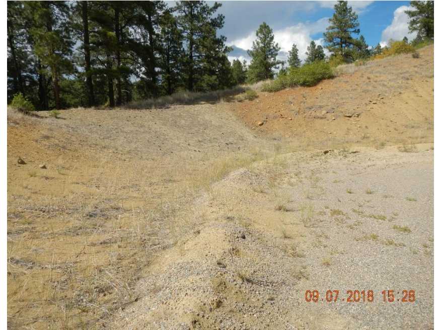
Run on control berm in northwest corner of location.
