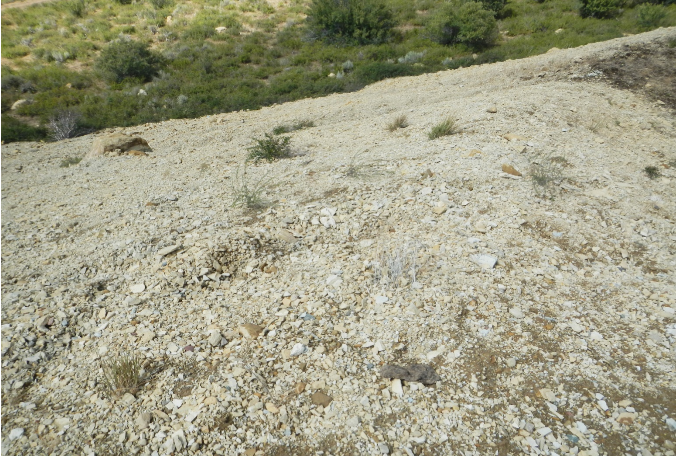
Photo#3: If seeding of Fill slopes was attempted it has been unsuccessful.
