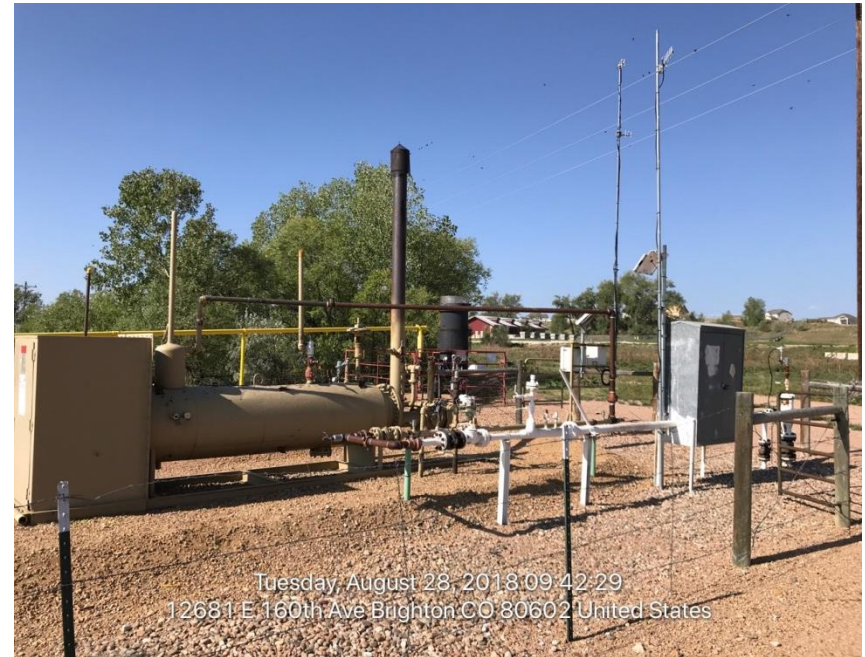
Photo#2 Separator/Gas Meter/ECD/Automation RTU
