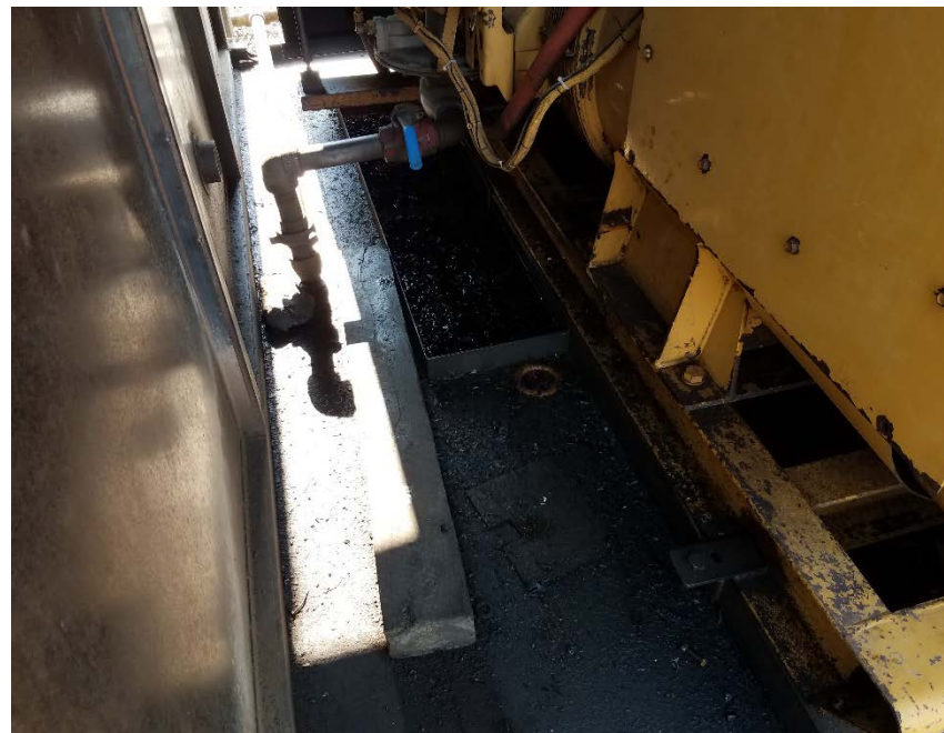
Location Photo #6, oil on floor of unit.
