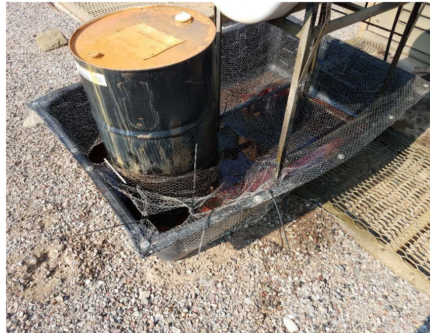
Location Photo #4, holes in wire, standing oil in catch pan.
