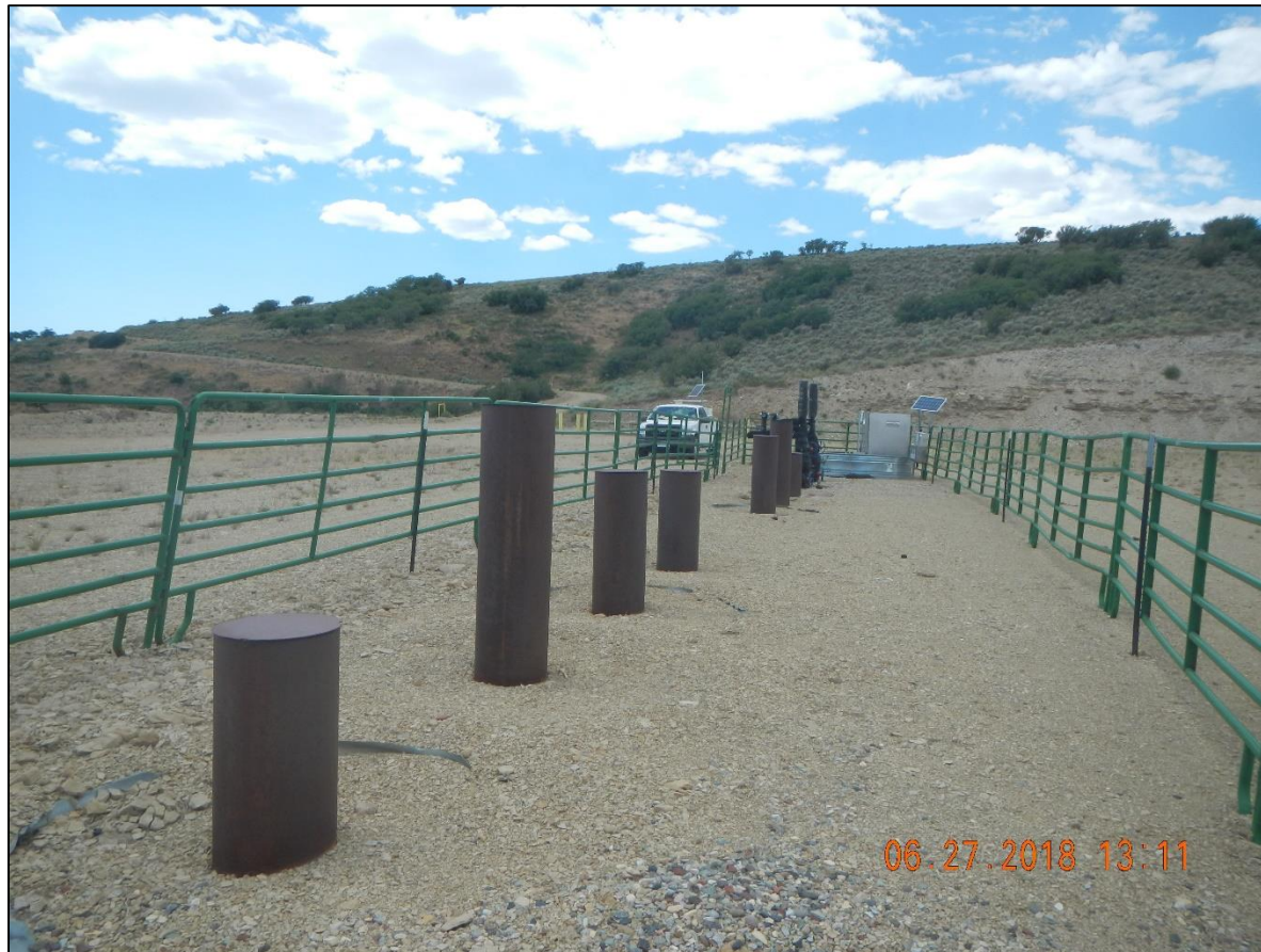
Seven conductors for undrilled wells
