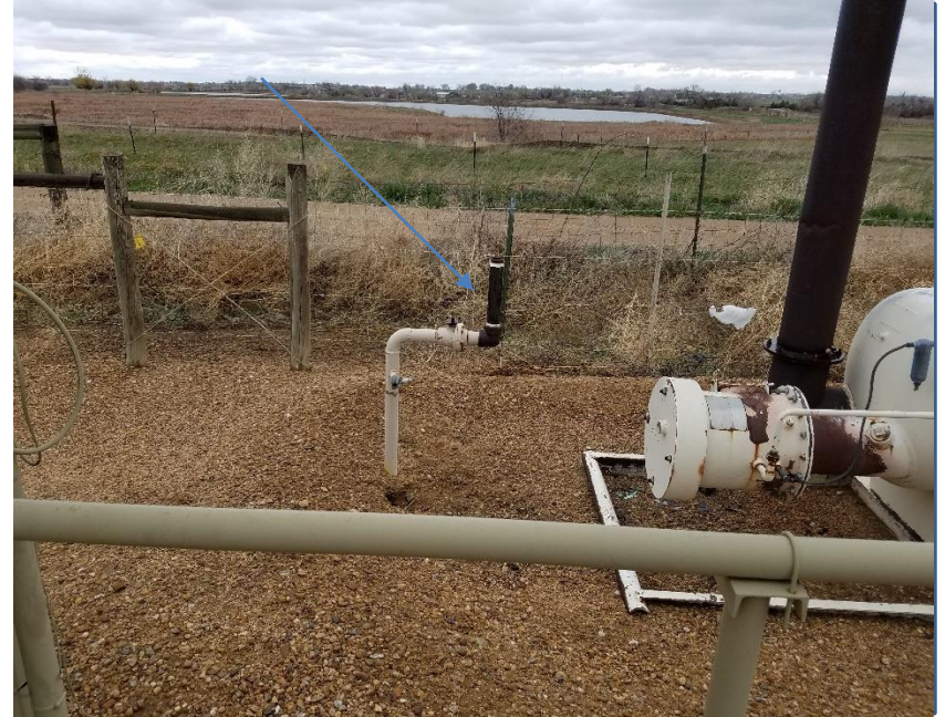
Photo 4. Unmarked riser no LO/TO
