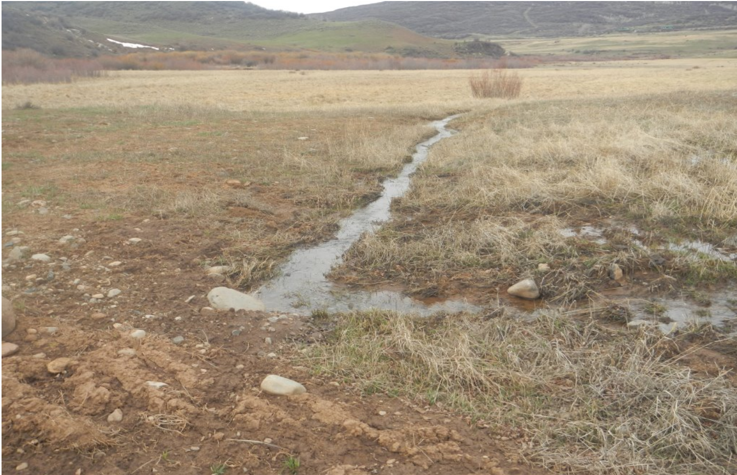
Photo#4: Existing ditches are diverting some of runoff water.
