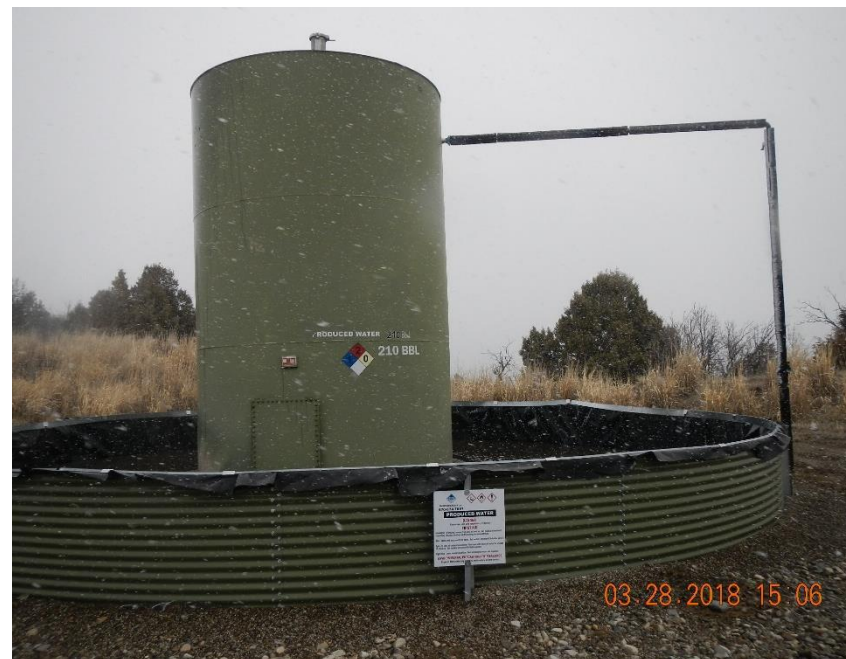
210 bbl. produced water AST with lined steel ring secondary containment.
