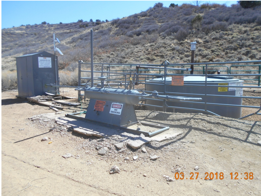
Meter housing with sign. Separator and tank
