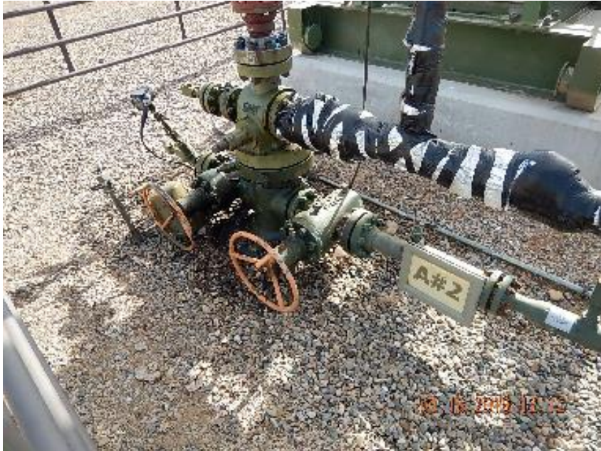
Photo 3: Impacted soil at A #2 wellhead.
