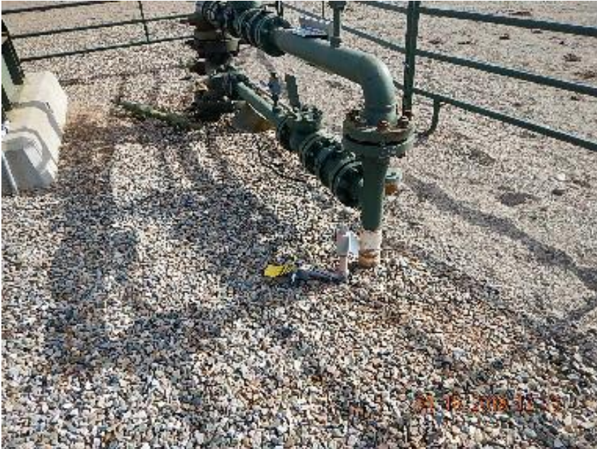
Photo 5: Unused riser at A #4 wellhead.
