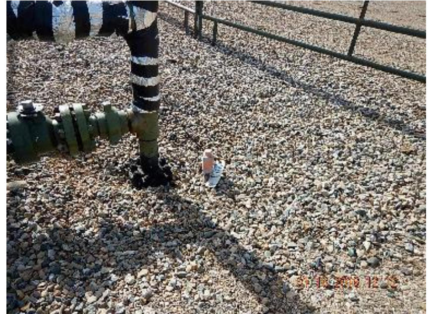
Photo 4: Unused riser at A #2 wellhead.
