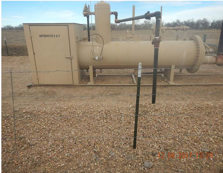
Photo 4: Separator is not properly anchored in floodplain.
