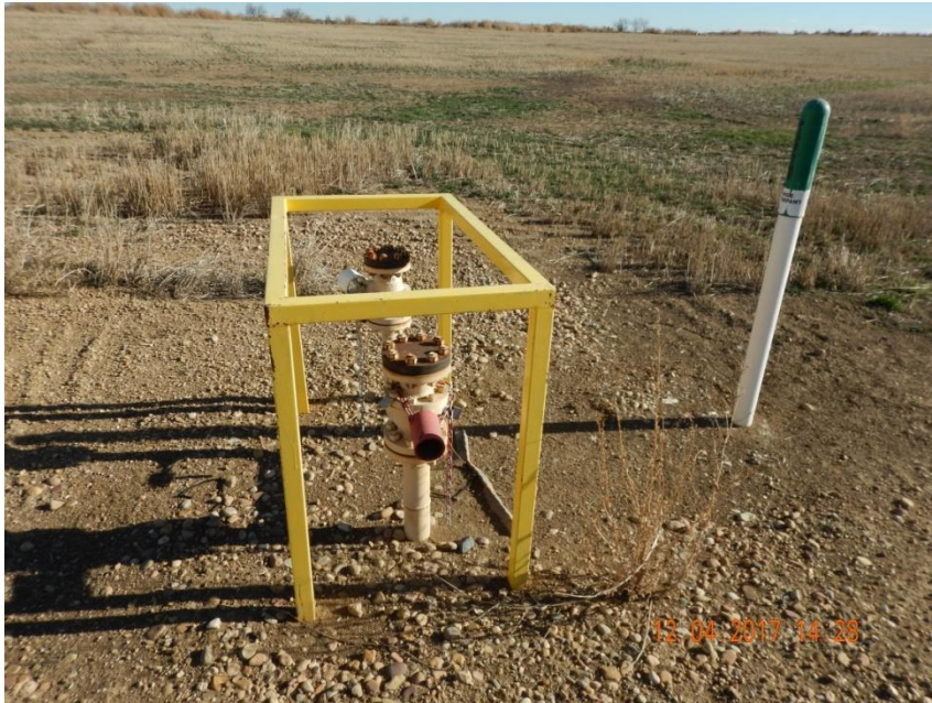
Photo 3. Photo taken from the southern battery location, facing East. Pipe risers remain at location. Operator needs to remove pipe risers per Rule 1004.a.
