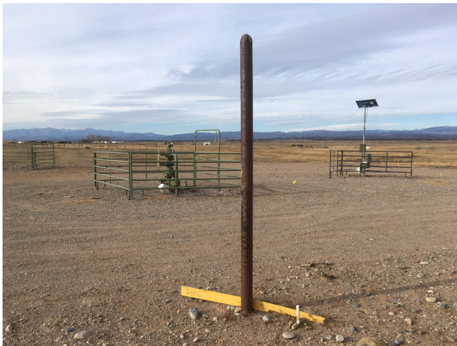
Photo 1. Simmons GU #1 plugged and abandoned well marker (1).
