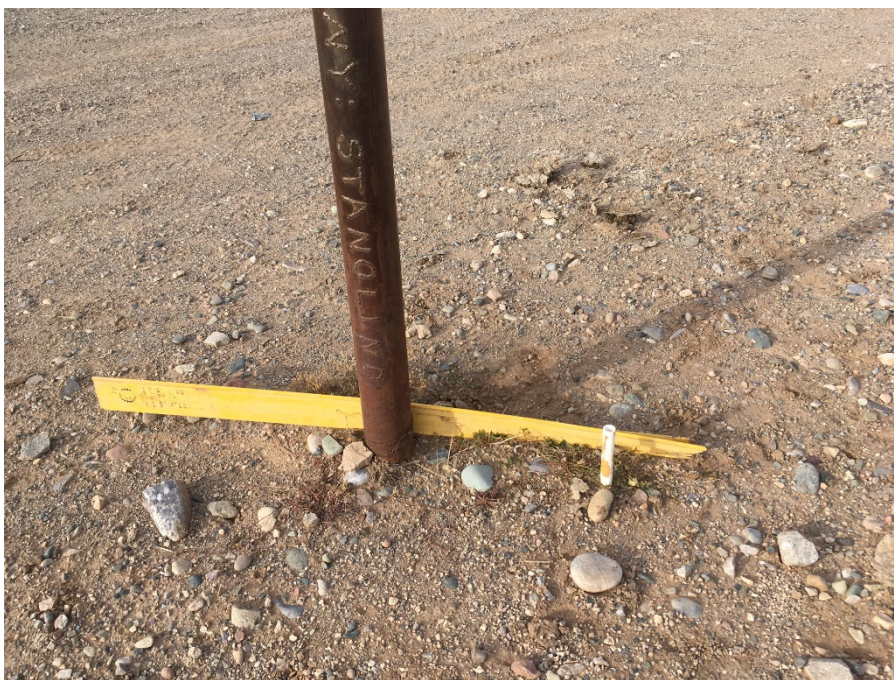
Photo 2. Simmons GU #1 plugged and abandoned well marker (2).
