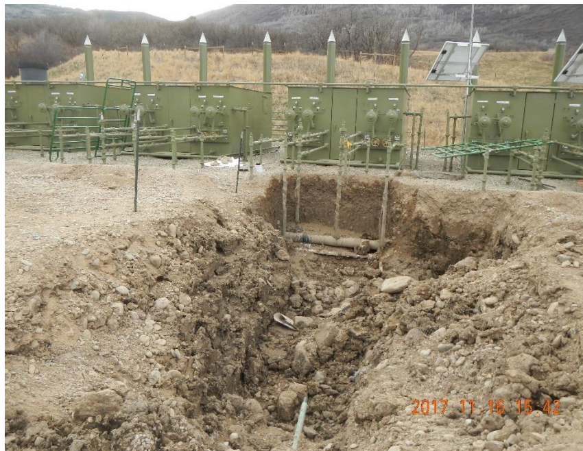
Looking west. Excavated area where the flowline from wellhead Rulison 23c-17 (API 045-18765) to the separator leaked.
