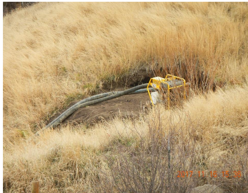
Pump to move water from retention pond back to the pad if necessary.
