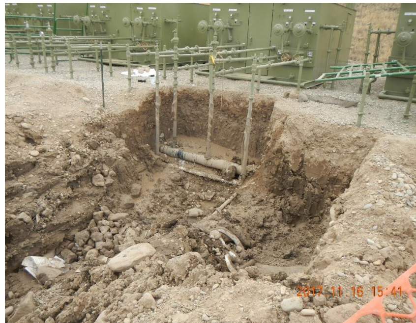
Excavation reached water table. A French drain crosses the excavation from left to right (south to north).
