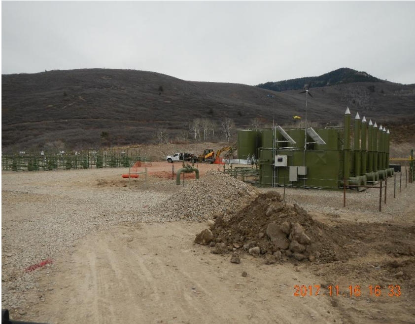
Looking south-southeast. Separators to the right, wellheads to the left and tank battery near the cut slope on the back.
