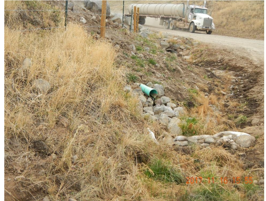
French drain (green pipe) discharging into the storm water drainage. Observe culvert further up. Water flows down to a retention pond (storm water BMP)
