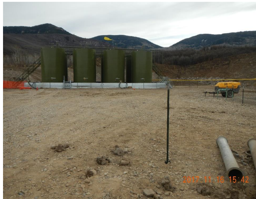
Looking south. Tank Battery, lined and bermed.
