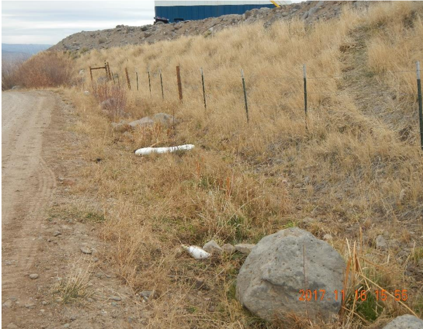
Storm water drainage with spill booms. Minimum if any staining was observed on booms.
