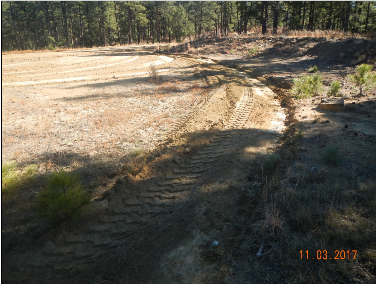
Photo 7. The diversion ditch was installed along the south side of the location.
