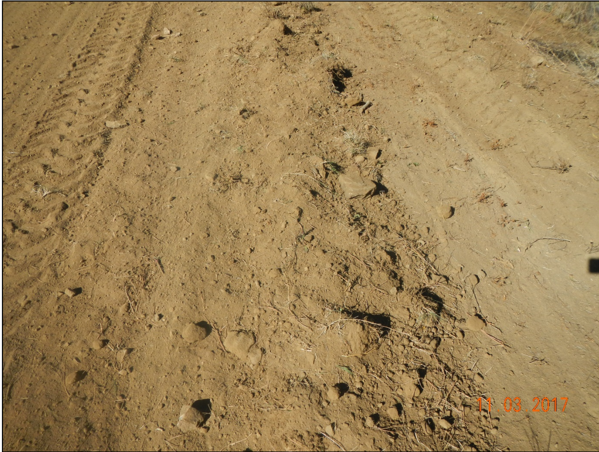
Photo 2. Soil was being pushed onto the road from the road side. The soil is loose and susceptible to erosion.
