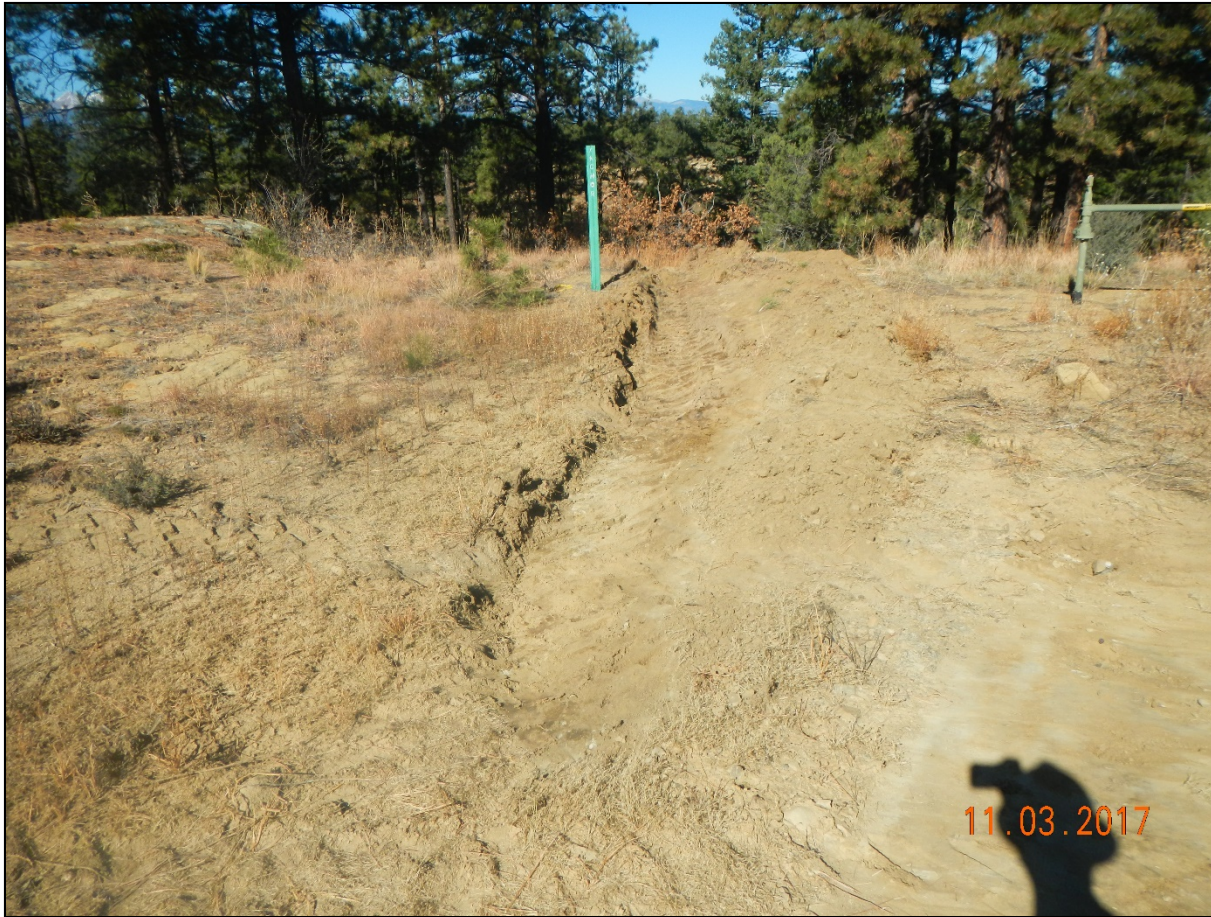
Photo 8. A diversion ditch was created for stormwater diversion. This disturbance is susceptible to erosion and no other BMP's are installed.
