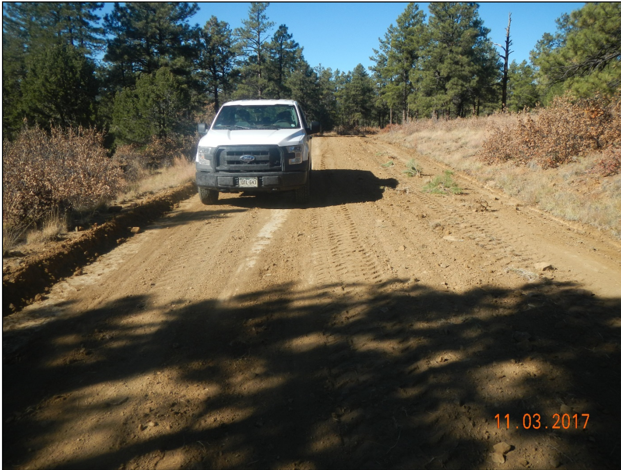
Photo 4. The vehicle shows the size of the access road. The road needs to be maintained to prevent widening of the rod.
