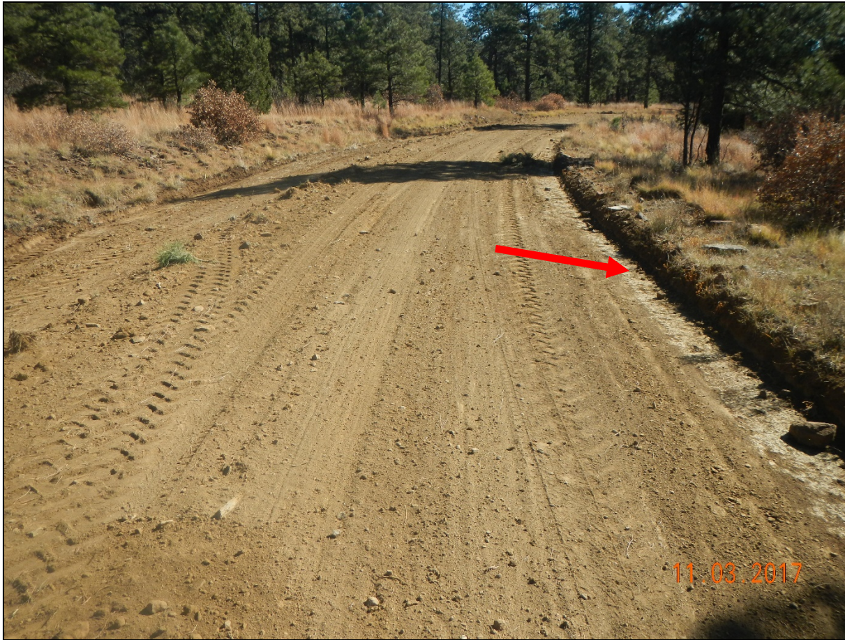
Photo 3. The arrow points to the side of the road where soil is being pushed onto the road which is also causing the road to become widened.
