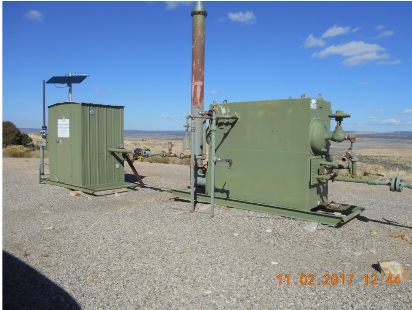
Meter housing, Separator
