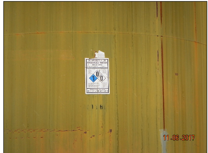
Photo 2. Update NFPA diamond for Fire Hazard or provide documentation for 0 rating. Capacity faded on tank.
