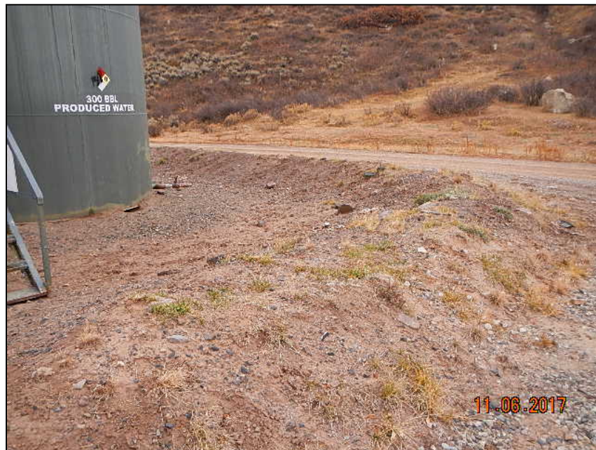
Photo 2. Vegetation and vegetation debris on berm and in tank containment. NFPA diamond starting to peel.
