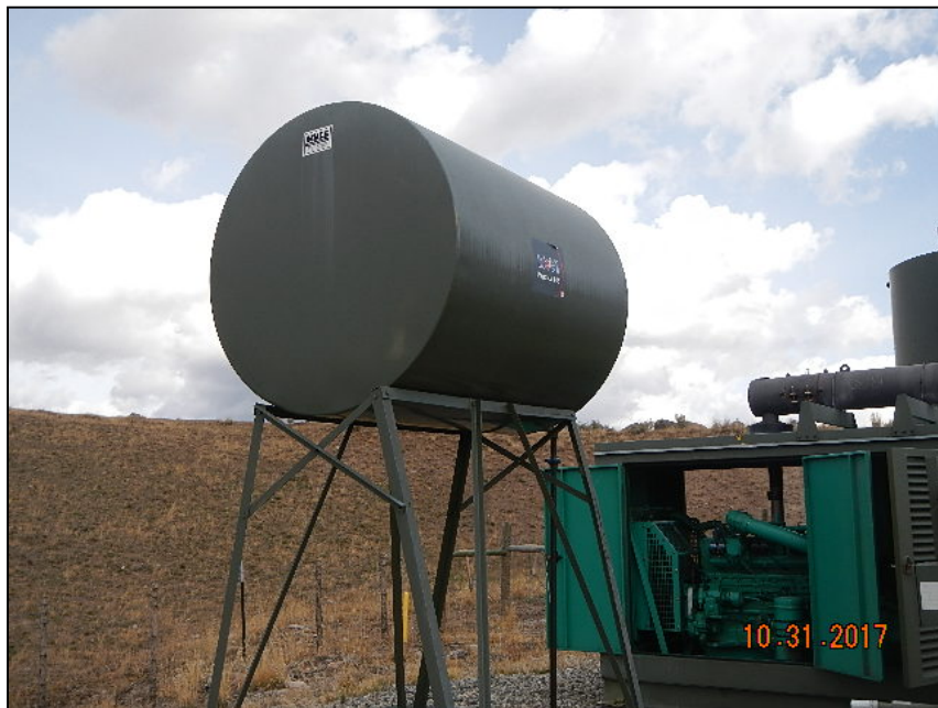
Photo 1. Oil tank with incomplete signage.
