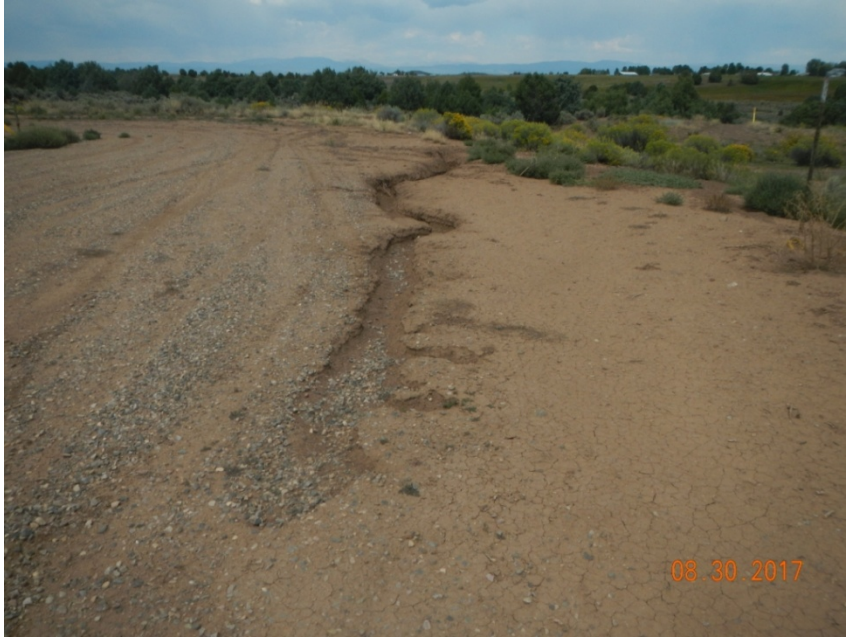
Photo 5: View of erosional channel approximately 2.5 feet wide and deep on the eastern edge of the working area.
