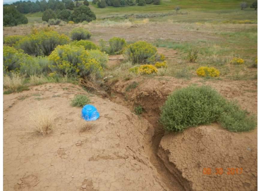
Photo 6: View of erosional channel downstream of Photo 5, in fill slope.
