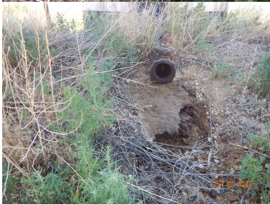
Photos 2 & 3 - Historical accumulations of oily waste at crude oil valves (top) and loadout (bottom). Note: loadout is outside of berm and lacks secondary containment device.
