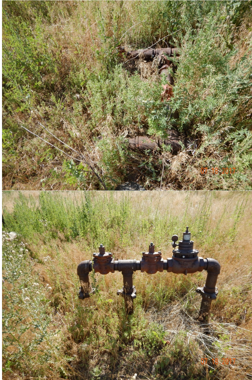
Photos 6 & 7 - Flowline risers/manifolds with valves located between tank battery and separator. Note: uncontrolled weeds.
