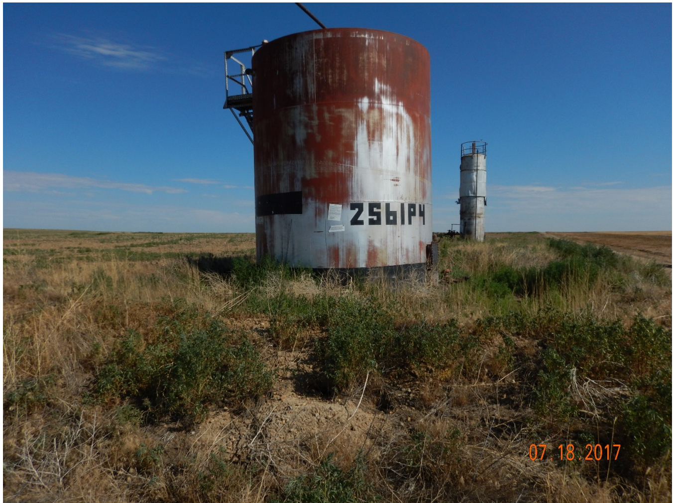
Photo 1 - Schmidt 1-B Tank battery. Note: tank lacking required labels/placard and earthen berms are overgrown with weeds.
