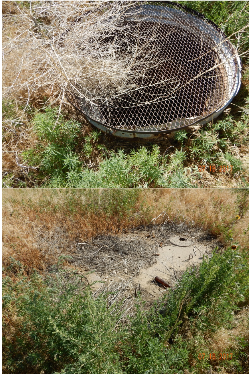
Photos 4 & 5 - Mesh-covered culvert (top) and buried cement vault (bottom) located north of crude oil AST. Note: culvert contains water and cement vault is overgrown. Facility ID #114389 was created for culvert in COGCC database.
