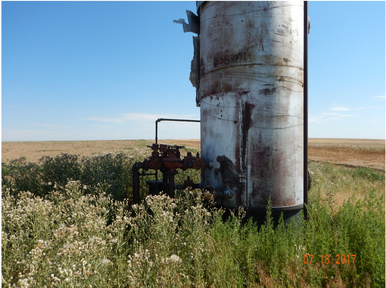
Photo 8 - Flowline riser assembly at vertical heater treater. Note abundance of weeds encroaching upon equipment.
