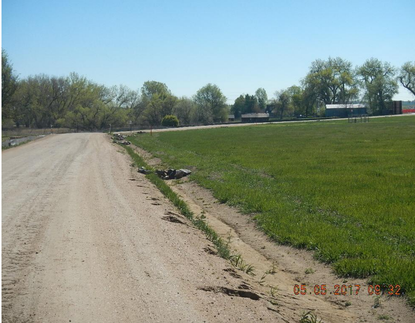
Ditch and stone check dams along access road
