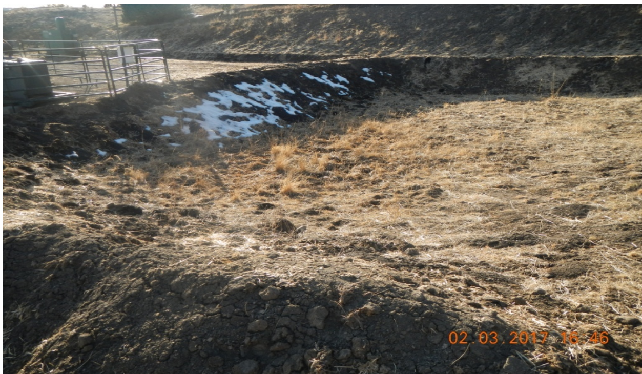
photo 2: Pit at the north side of the location. No free board marker was noticed.
