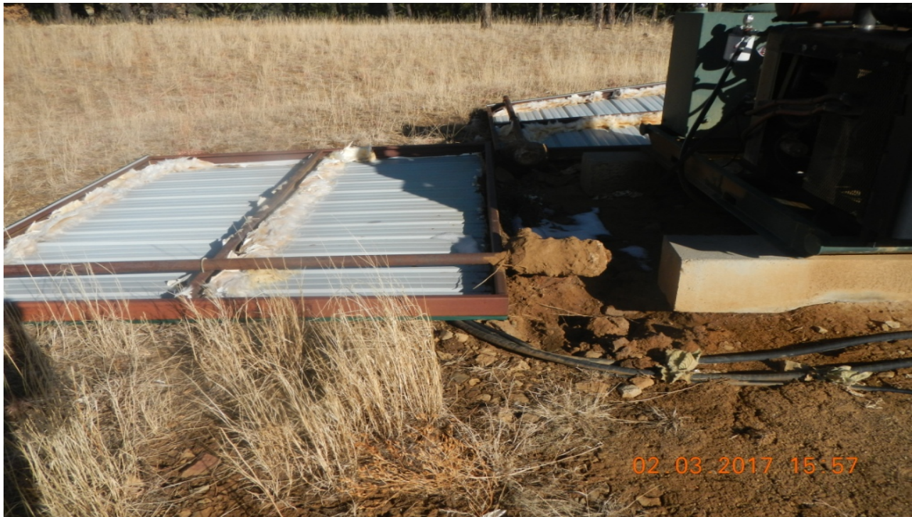
photo 3: The sound walls have fallen over.
