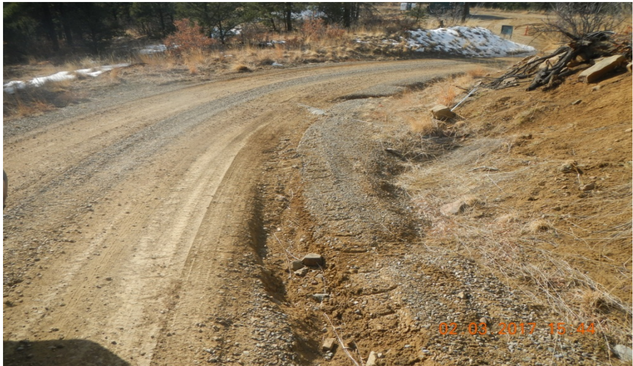
photo 1: There are signs of erosion along the access road near the location. Stormwater is not being directed toward the culvert.
