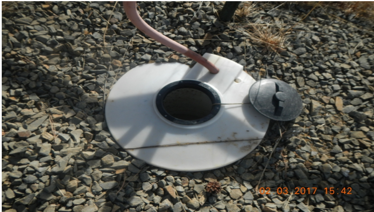
photo 7: The lid was left off the buried container at the east side of the location.
