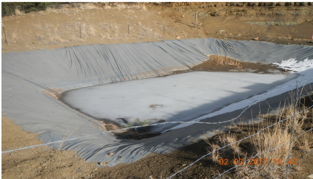
photo 5: Lined pit at the northeast side of the location.
