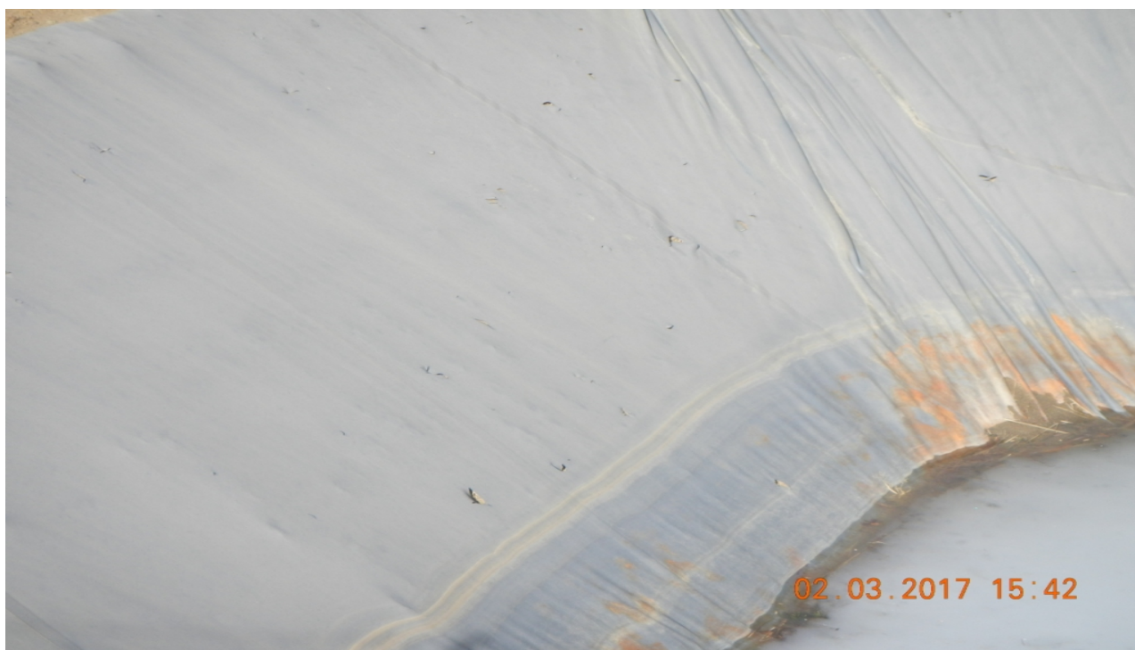
photo 6: There appears to be tears in the pit liner.
