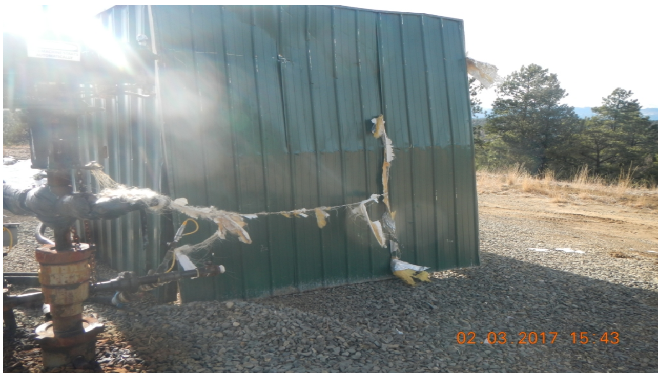
photo 8: The insulation is outside of the sound wall near the well head.
