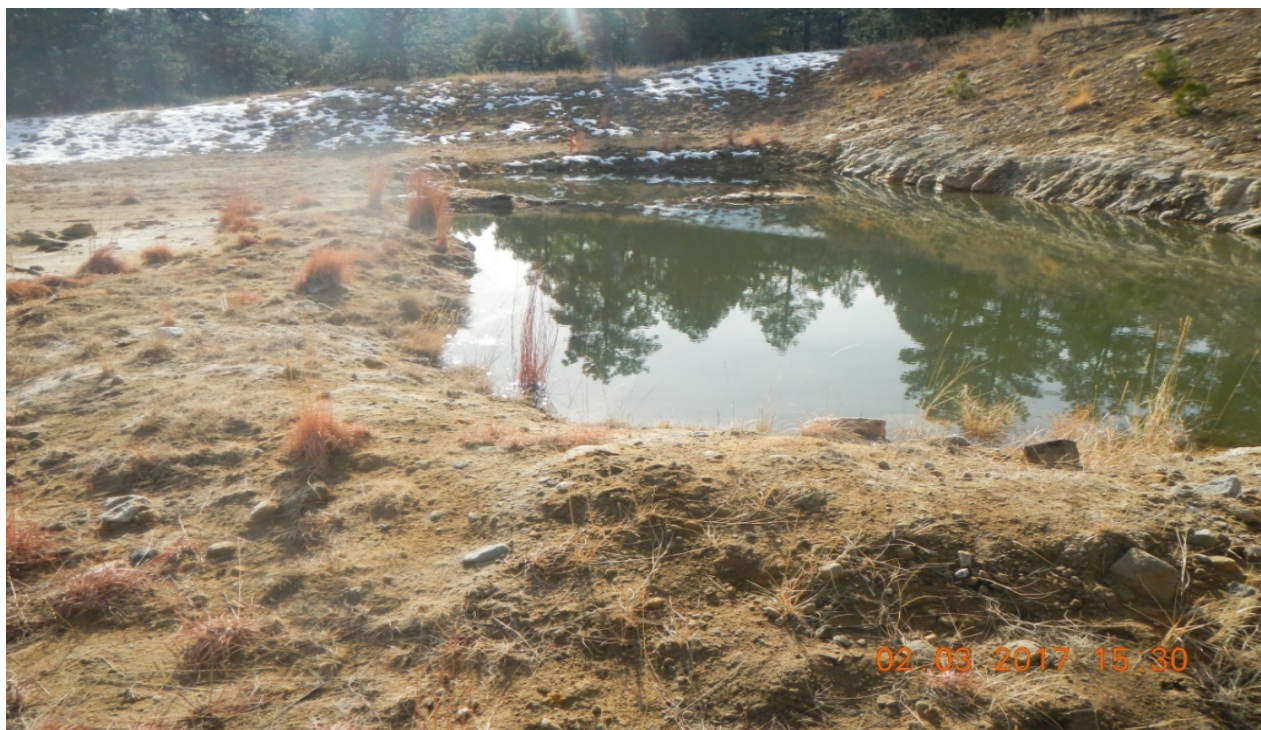
photo 2: Pit at the northwest side. The pit did not appear to have 2 feet of freeboard.
