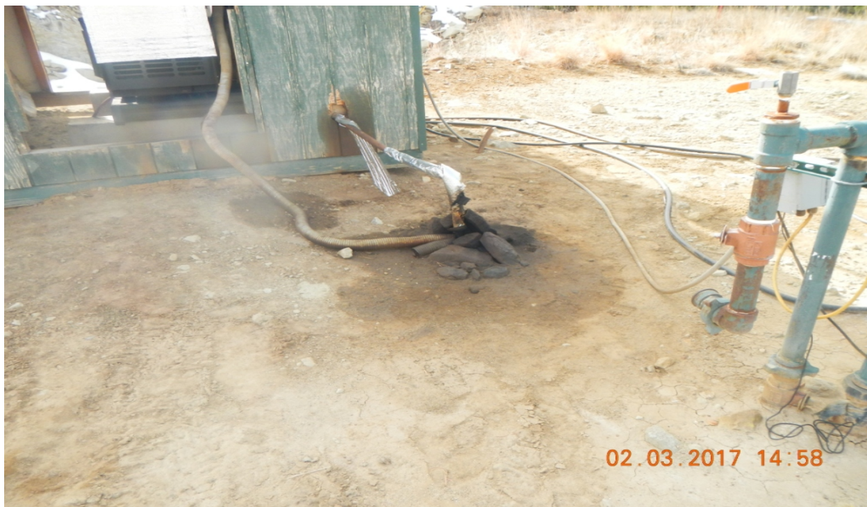
photo 5: There is stained soil around the exhaust from the engine.
