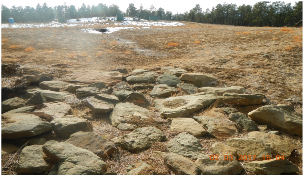
photo 8: East side of the location facing southwest. Rock rip/rap is placed at the drainage.
