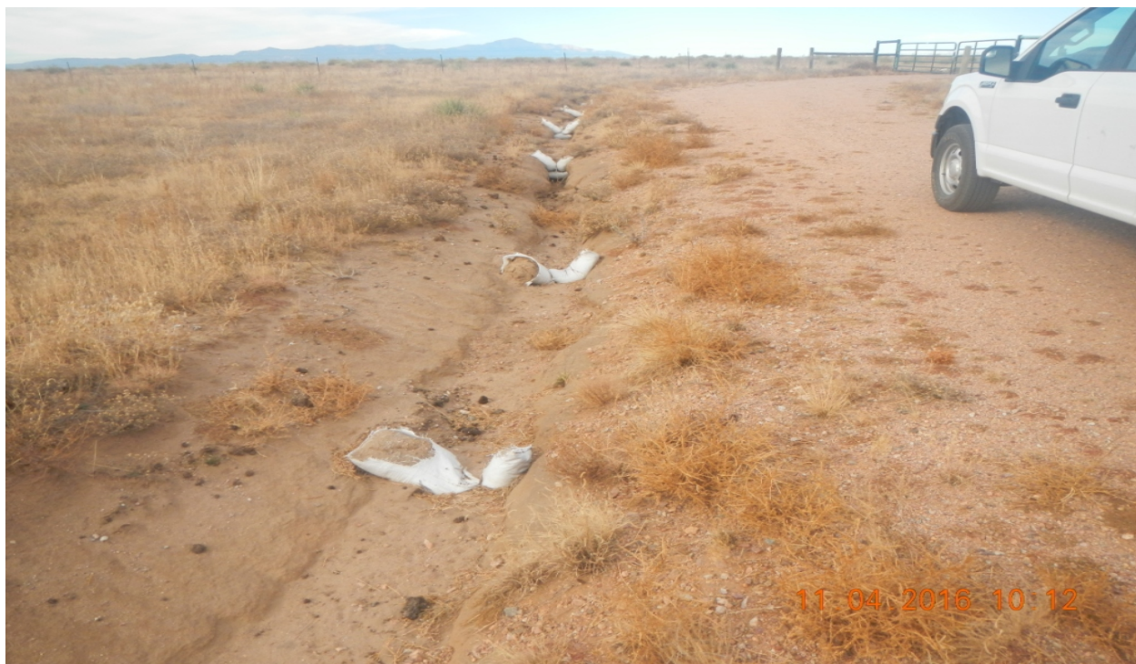
photo 1: Facing west along the access road. This erosion channel was documented in the previous inspection.
