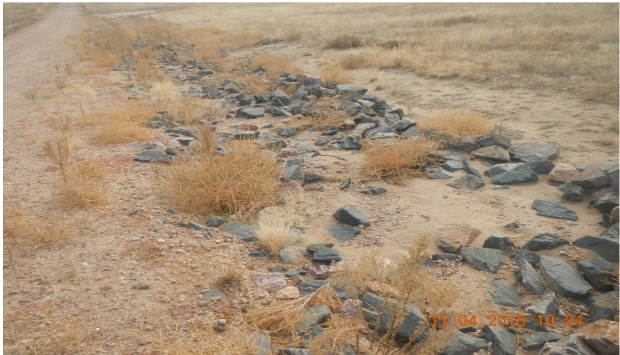
photo 8: Facing back towards the east along the access road where rip/rap rock has been placed.
