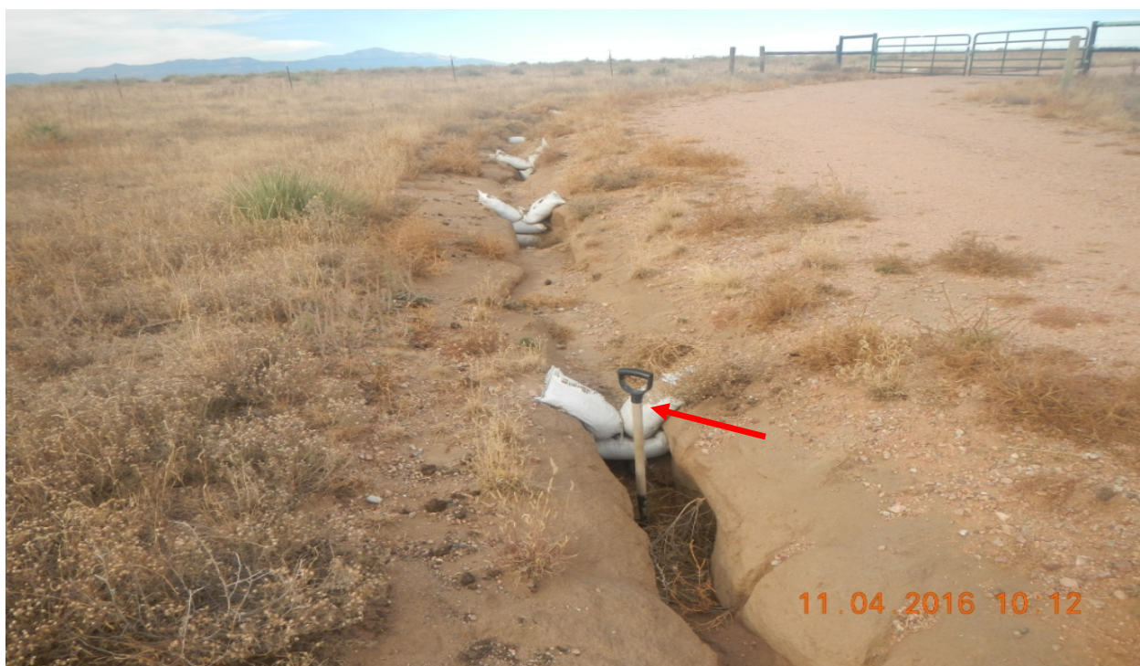
photo 2: A 3 ft. shovel indicates depth of channel.
