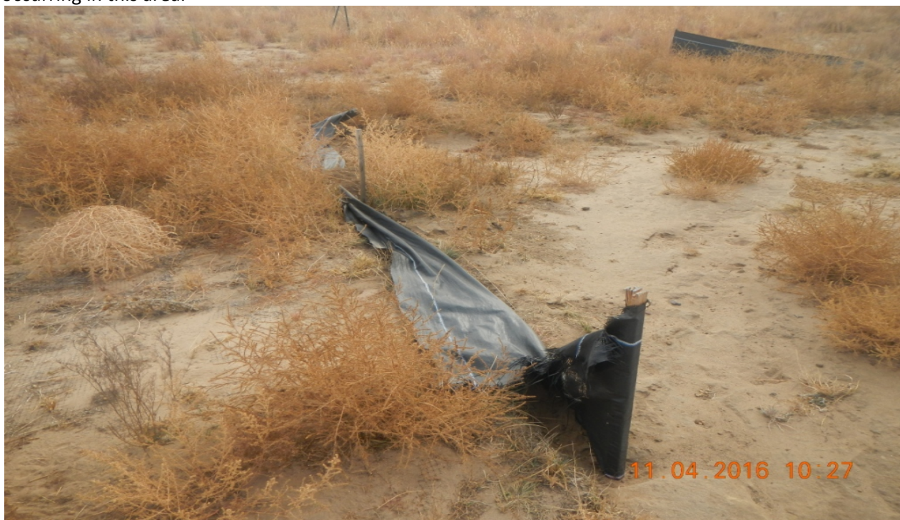
photo 12: The sections of silt fence are in disrepair.
