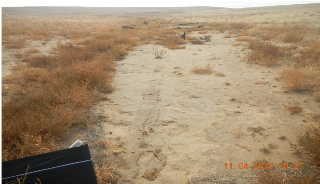
photo 11: Vegetation in areas near the silt fence sections has not established. There are signs of erosion occurring in this area.
