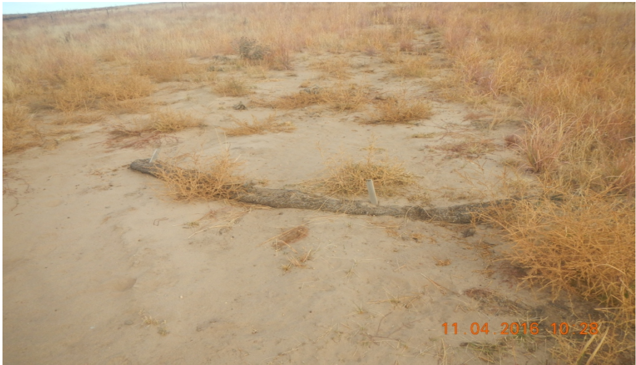
photo 15: There are wattles which are filled in with sediment.
