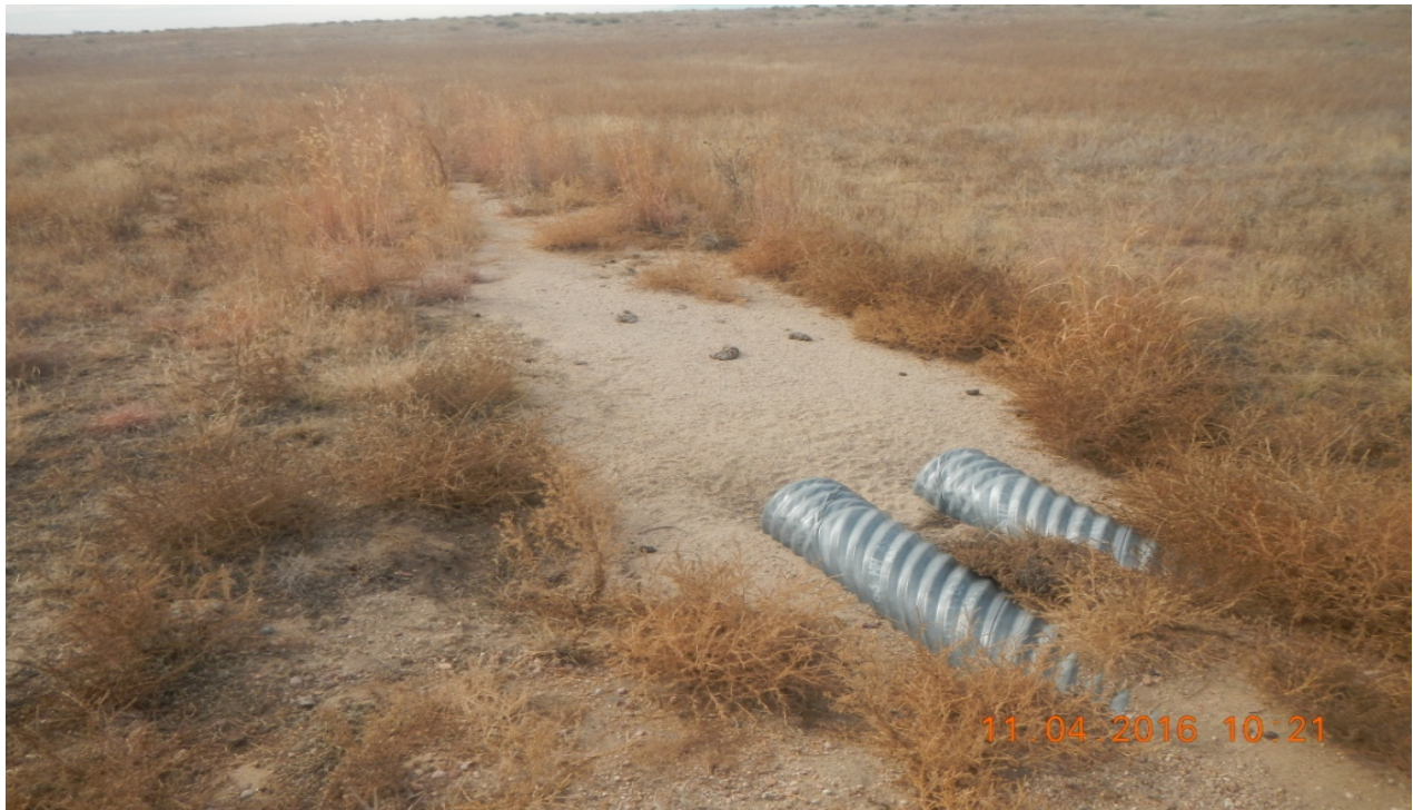
photo 5: Sediment is being directed out into the pasture and is beginning to fill in the culverts.
