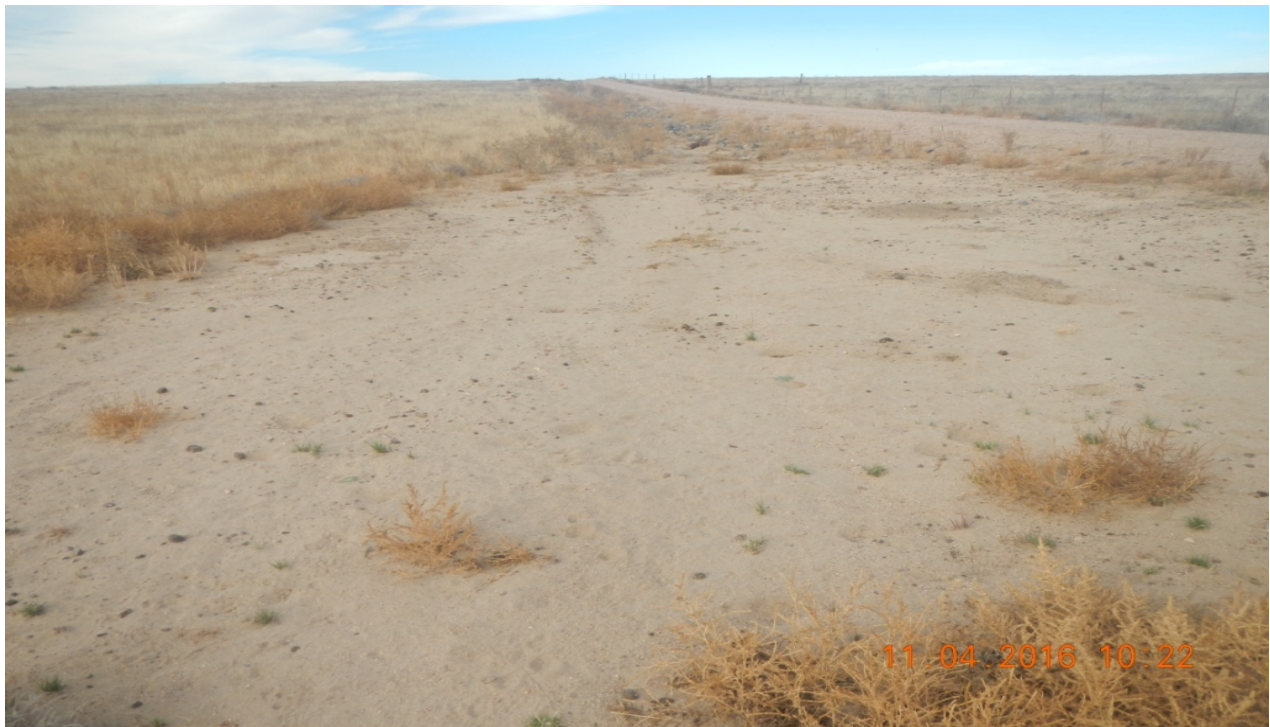
photo 6: Facing west at the south side of the access road. Sediment appears to have deposited from erosion off the access road.
