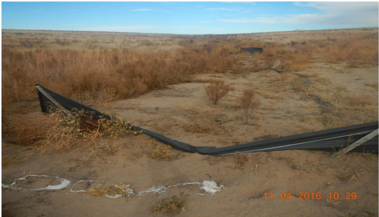
photo 16: Facing north at the location. The white sandbags are filled in with sediment and the sections of silt fence are in disrepair.
