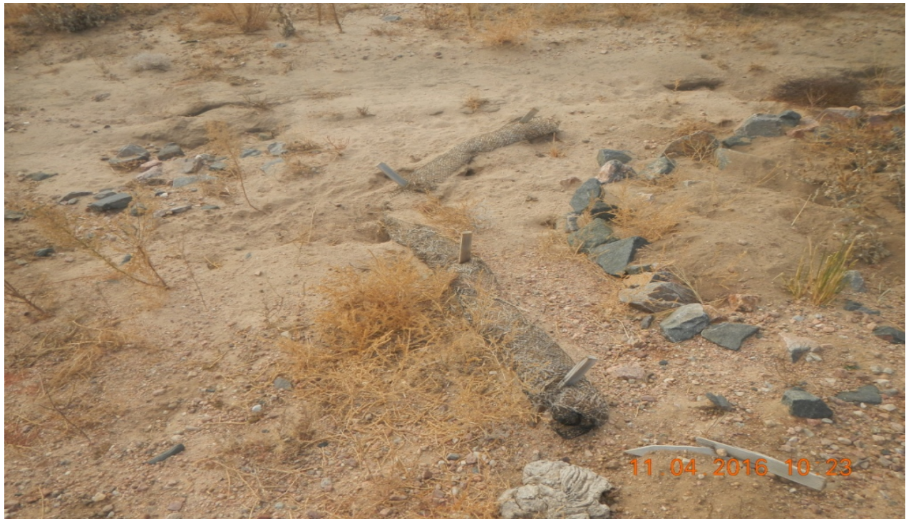
photo 7: Wattle placed at the end of the rip/rap along the access road is filled in with sediment.
