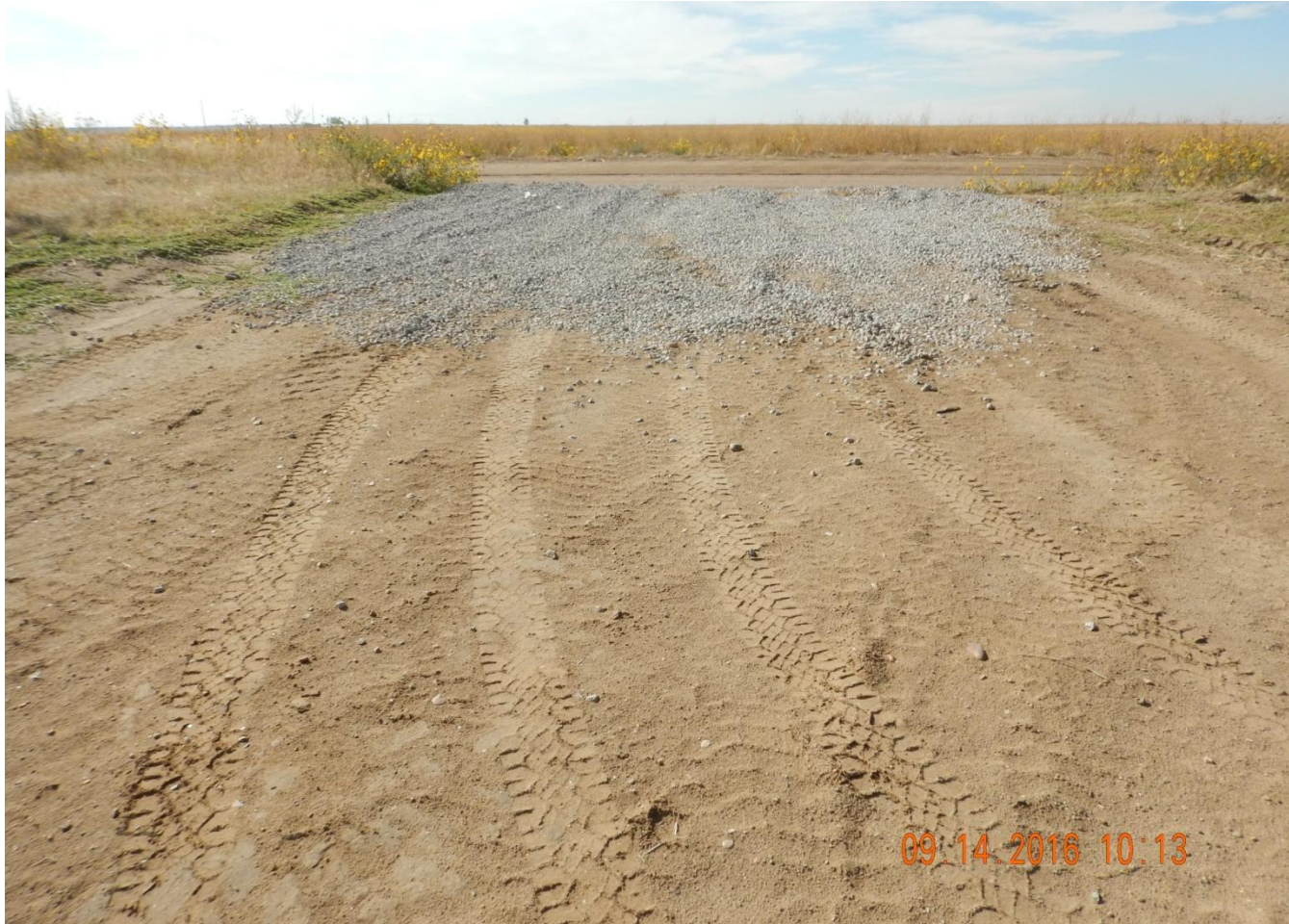
Photo 5. Photo taken from the eastern entrance, facing South. Gravel installed at location entrance.
