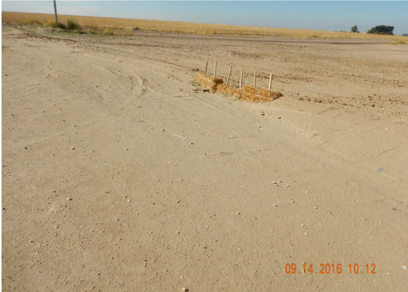
Photo 1. Photo taken from the western location, facing Southwest. Berm was constructed and straw bales installed to control sedimentation from leaving location.
