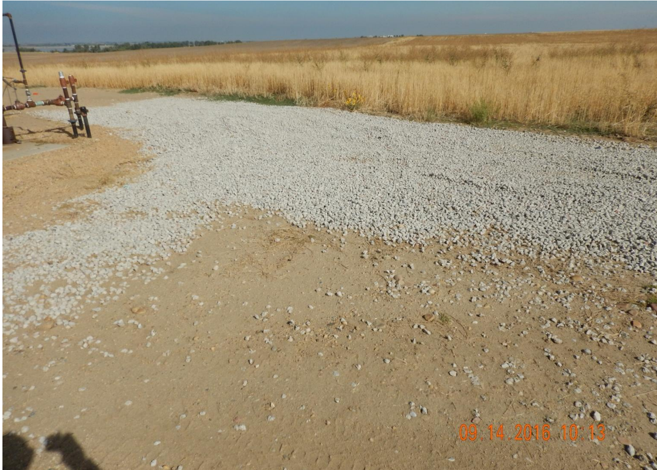
Photo 4. Photo taken from the northern location, facing Northwest. Gravel installed to stabilize location and prevent erosion.
