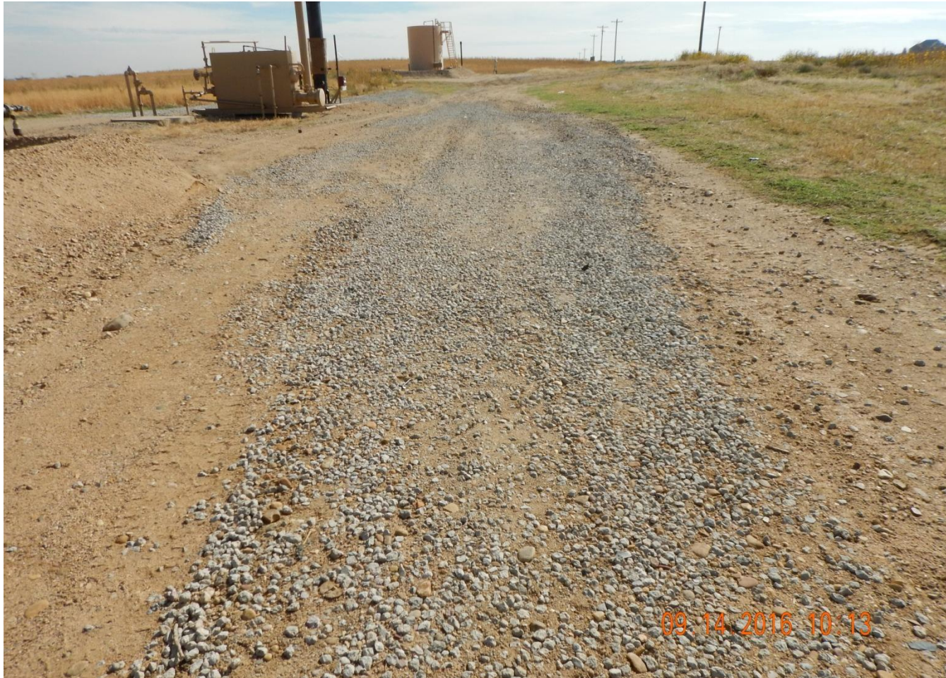
Photo 3. Photo taken from the western entrance, facing East. Gravel installed to stabilize location and prevent erosion.
