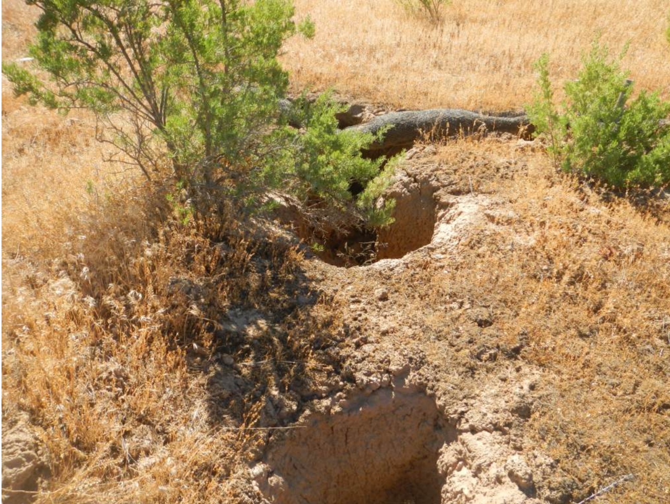
Photo#9: Water is undercutting wattles at multiple sites.
