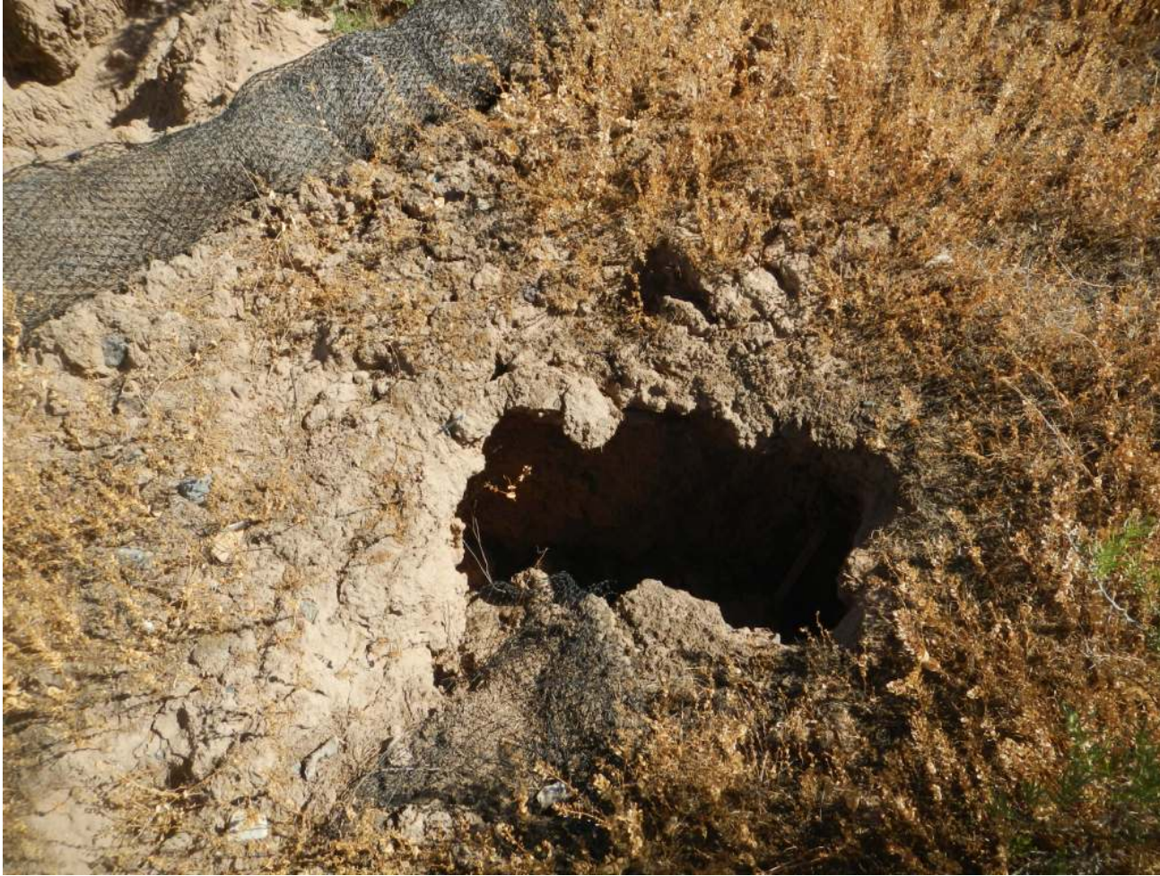
Photo#8: Water is undercutting wattles at multiple sites.
