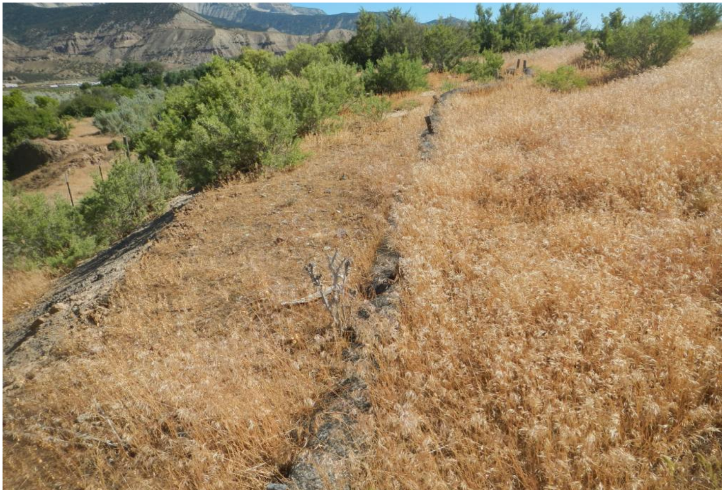
Photo#7: Wattles running East to West at NW perimeter of Location
