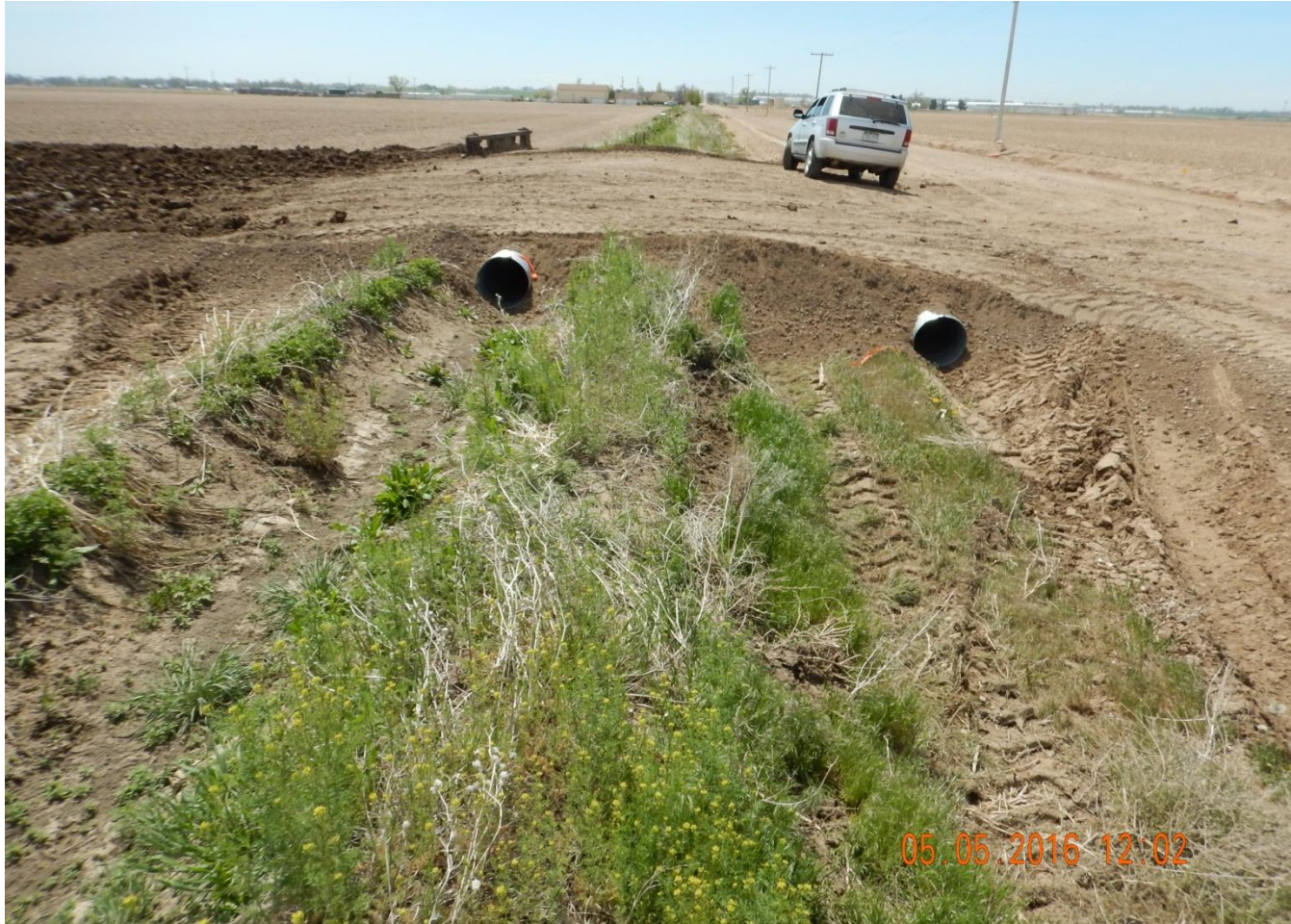
Photo 1. Photo taken from entrance of location, facing South. Culverts installed at entrance.
