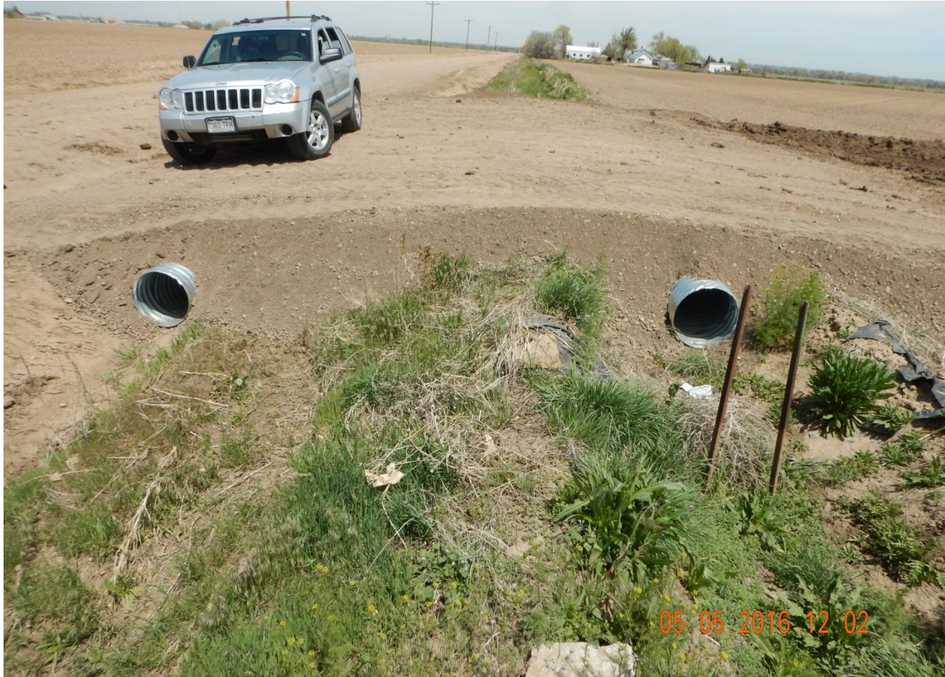
Photo 2. Photo taken from entrance of location, facing North. Culverts installed at entrance.
