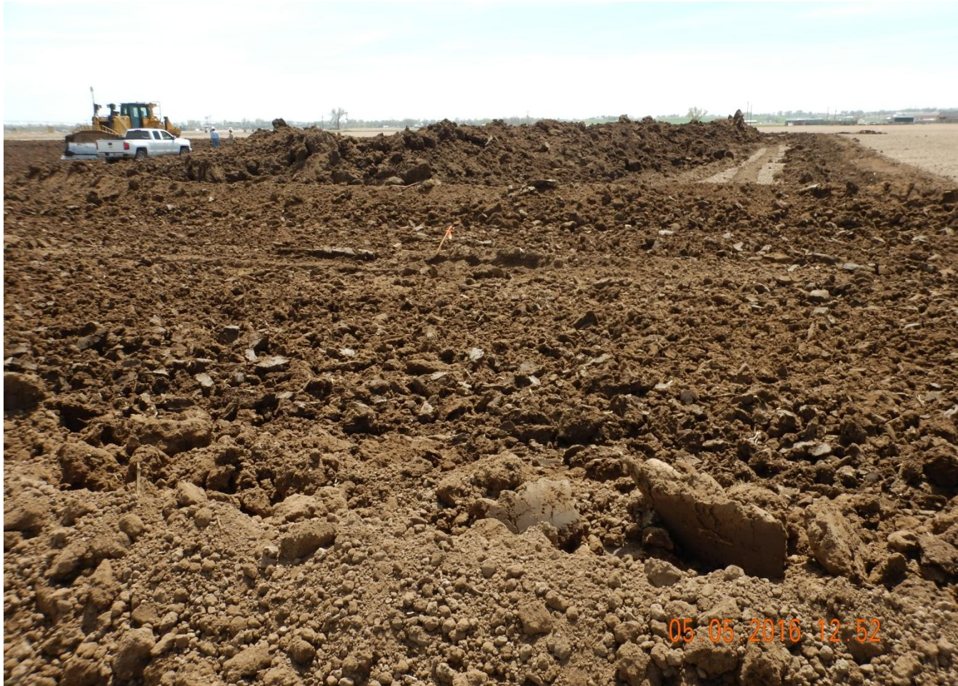
Photo 9. Photo taken from northwest location, facing South. Topsoil stockpile in center of photo. Topsoil stockpile needs to be stabilized upon completion of salvage process.
