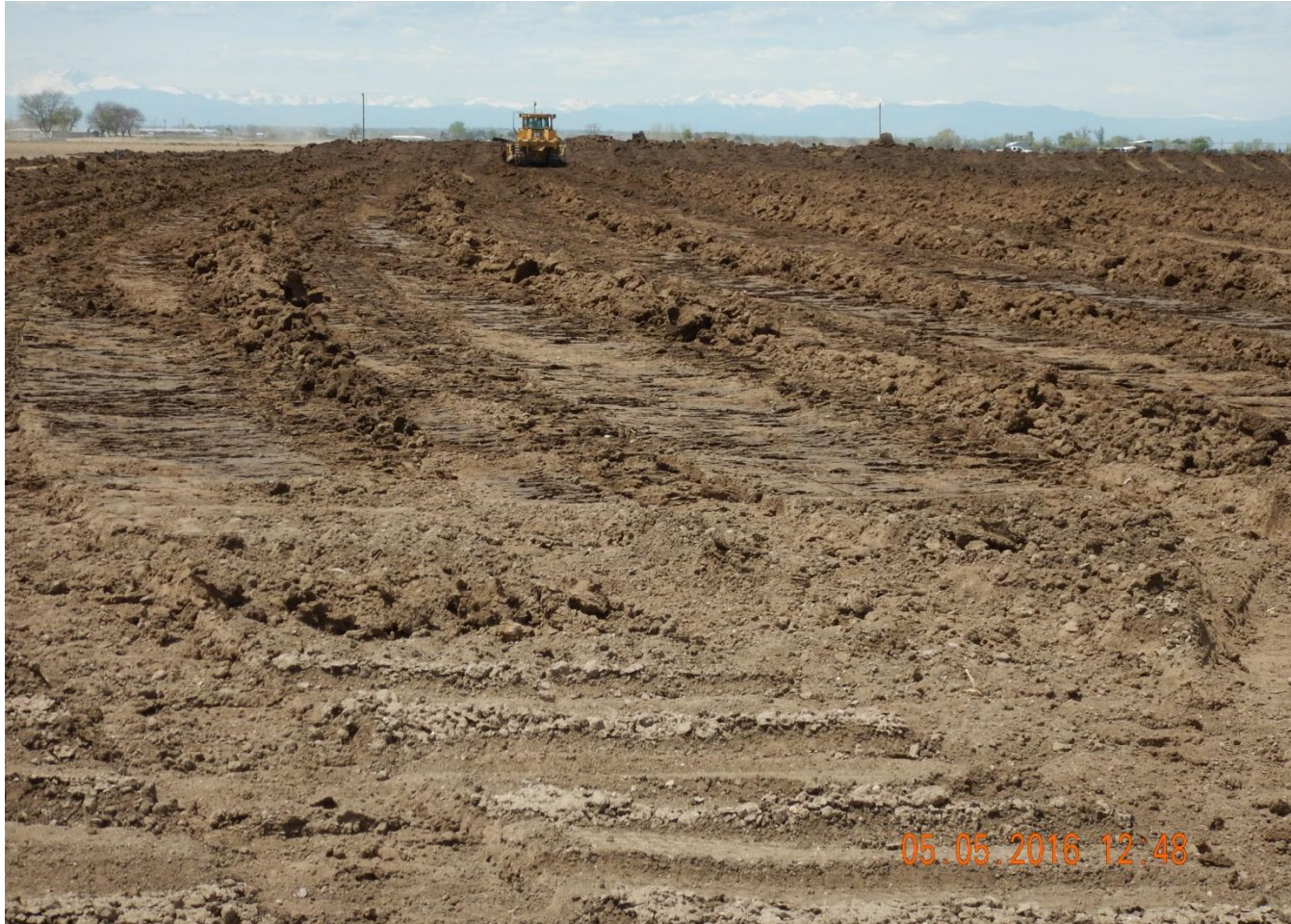
Photo 8. Photo taken from eastern location, facing West. Topsoil salvage in process.
