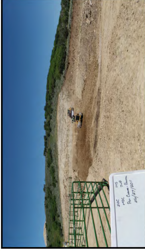
Photo 6 – Pit during backfilling operations.
