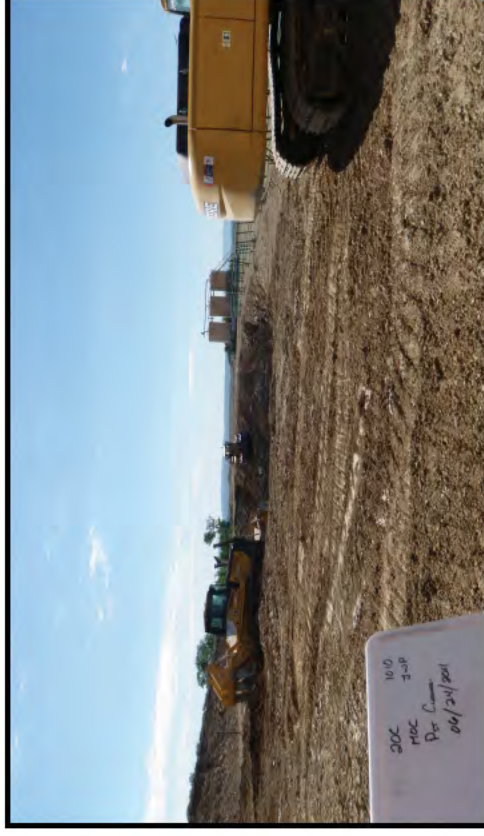
Photo 4 – Roller and D8 rolling and mixing material in the pit.
