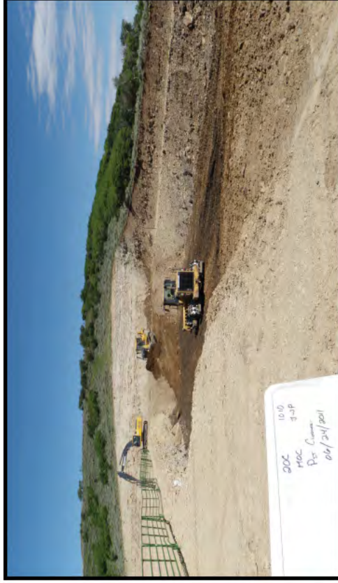
Photo 3 – Roller and D8 rolling and mixing material in the pit.
