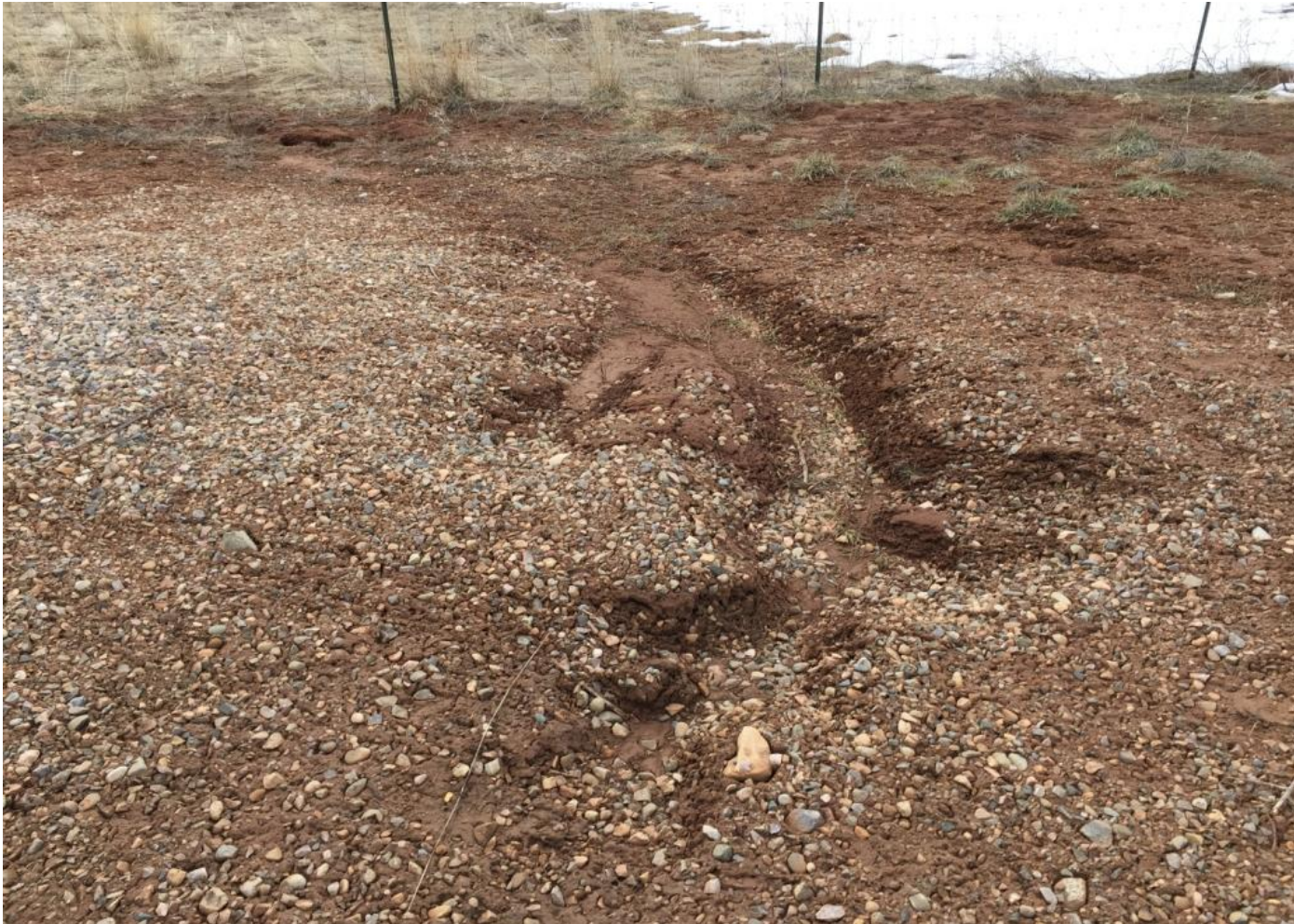
Photo 1. View of stormwater erosion channel forming in southwestern portion of the project area. Channel is approximately 12 inches wide and deep.
