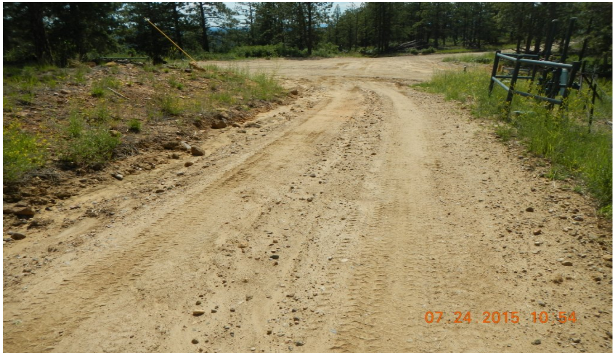
photo 3: Facing east back towards the main road. It appears sediment is being transpoted down towards the main access road.
