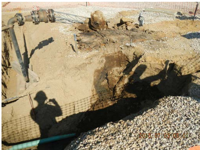
Compromised line leaking fluids and gas.
