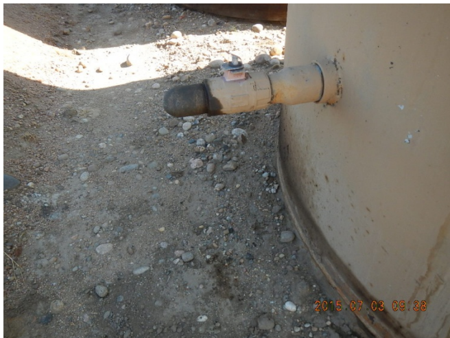
Leaking fittings. Tank Number 54023.
