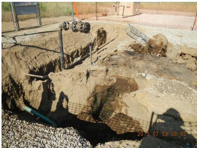
Compromised line leaking fluids and gas.
