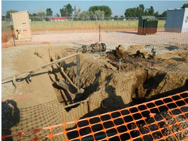
Footprint of where meter shed was located. Stained soil.
