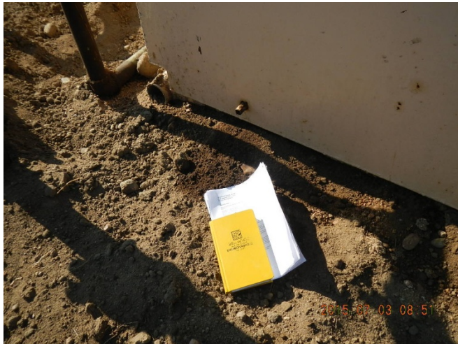
Oily soil beneath line.
