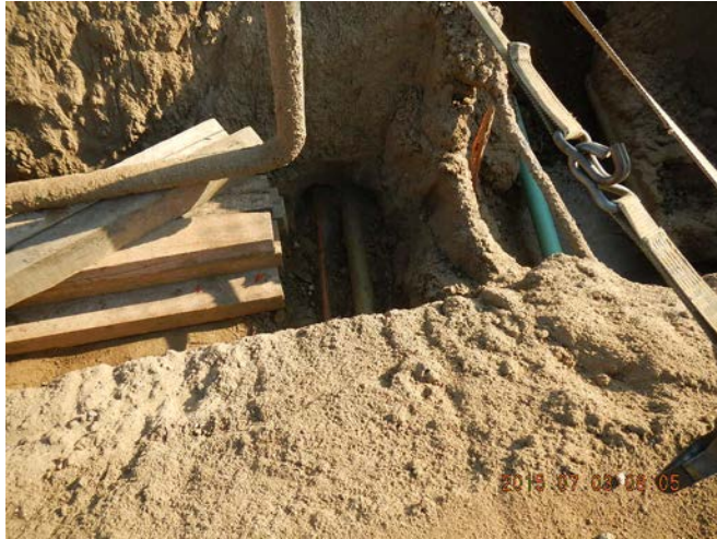
Texas Tea flowlines immediately to the right of wood cribbing.
