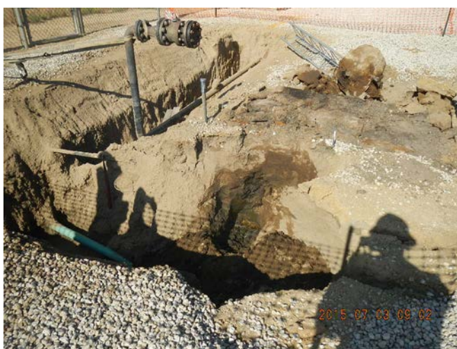
Compromised line leaking fluids and gas.
