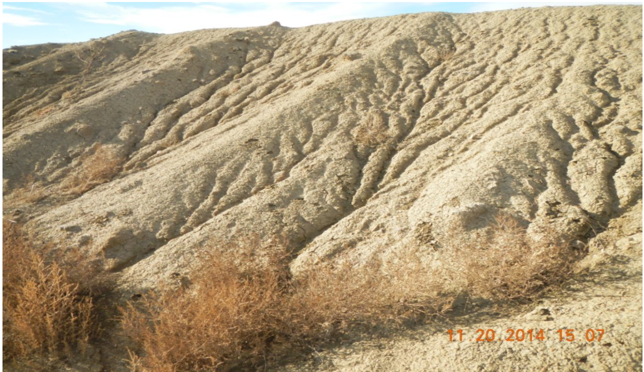
photo 4: Top soil stockpile is being eroded and is not being protected from degradation.
